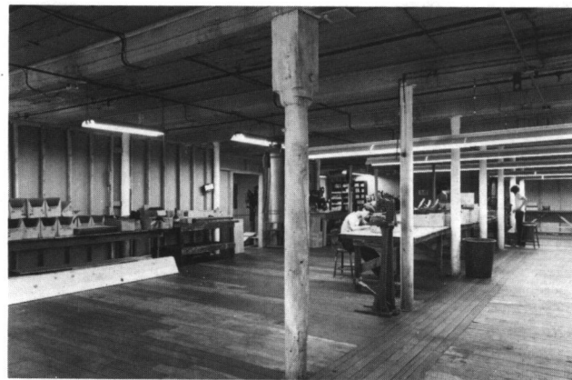
Fig. 53: Interior, Dyerville Mill (1830); 610 Manton Avenue. Showing use of heavy wooden columns, developed as a fire retardant.
