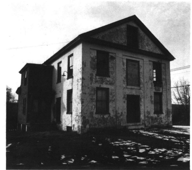
Fig. 52: Commissary Building, Allendale Mill (c. 1822); 494 Woonasquatucket Avenue. The mill displays simplified Greek Revival details.
