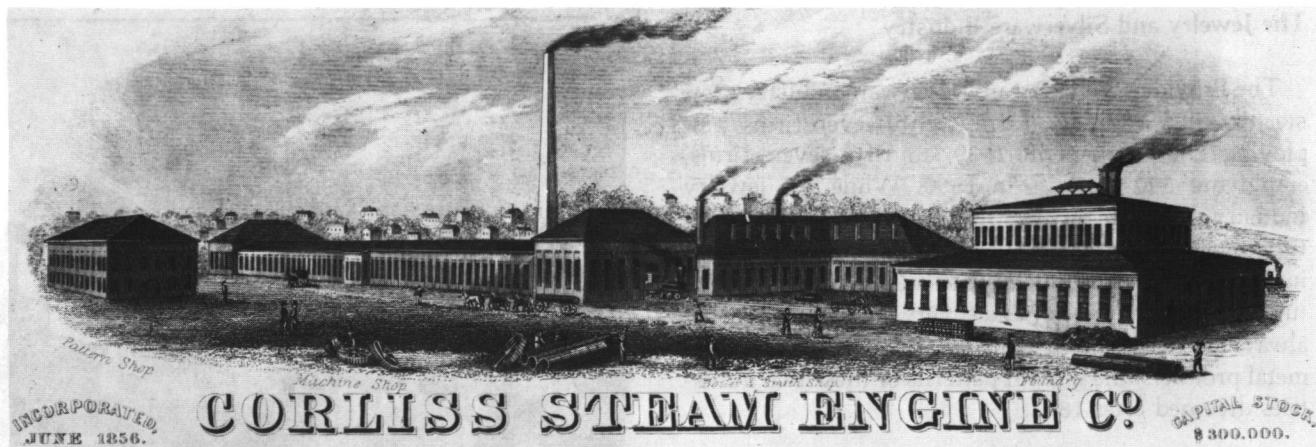
Fig. 13: Corliss Steam Engine Co. (c. 1857; buildings now altered); 14 West River Street; photograph c. 1857. Designed by George H. Corliss.
