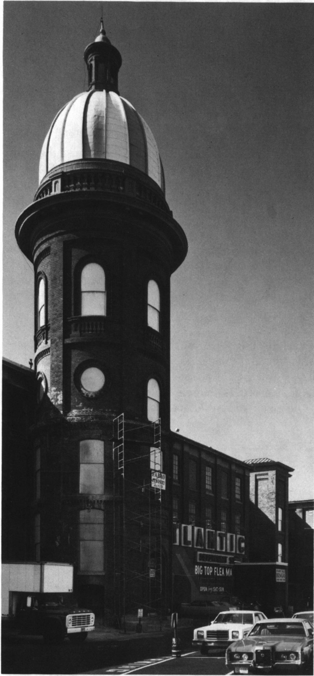
Fig. 64: Atlantic Mill (1863 et seq.). The round, paired towers are unusual, but the high domes on balustraded attics are formally kin to those on contemporary gasometers.
