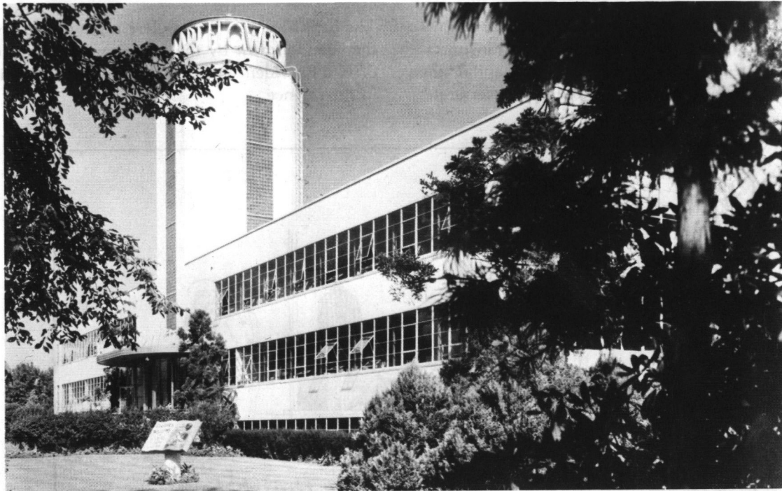
Fig. 47: California Artificial Flower Co. (1939); 400 Reservoir Avenue. One of the few Art-Deco industrial buildings of the era.
