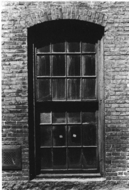
59b. Window detail with segmental arch.
