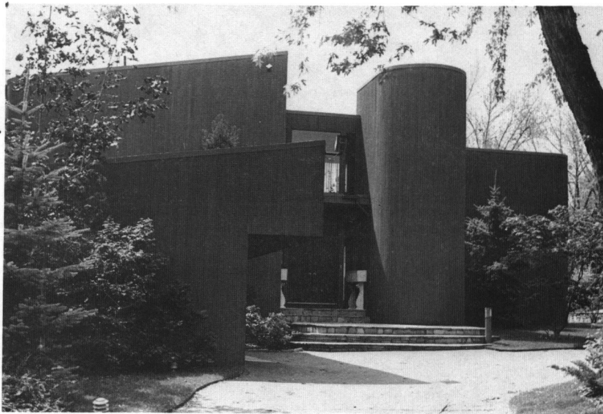
Joseph P. Esposito House (1974-75), 2 Woodland Terrace. Modern house inspired by design for California's Sea Ranch Condominiums.
