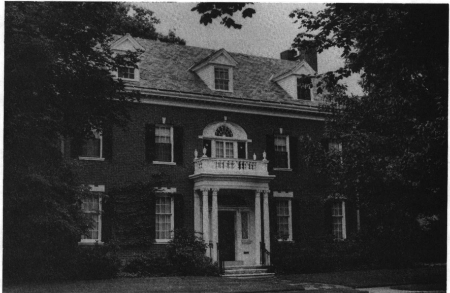
Robert L. and Caroline S. Gilman House (1930), 730 Elmgrove Avenue. Neo-Georgian house with Federal Revival detail.
