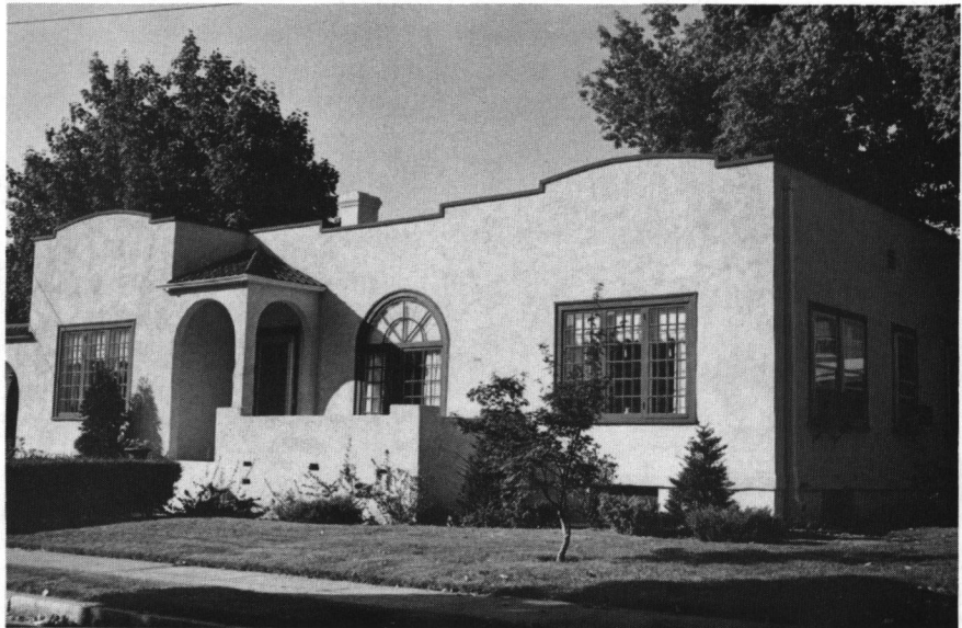
John B. and Rebecca Olevson House (ca. 1926), 30 Elmway Street. Spanish Colonial Revival bungalow.
