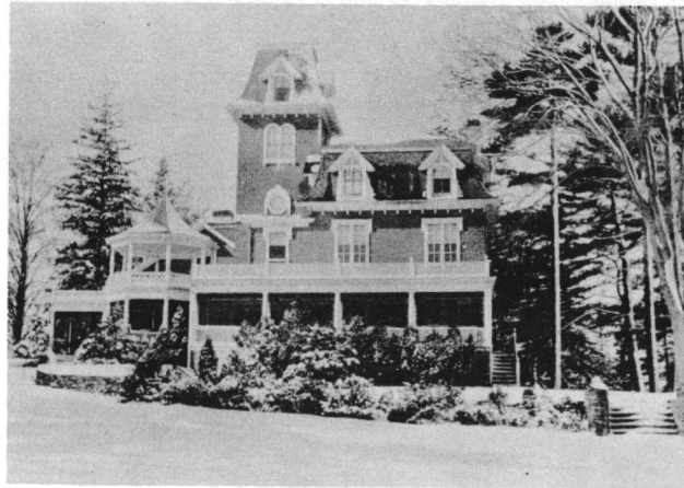
Fig. 50: Quidnessett Country Club, former Wightman-Allen-Knight House (mid-18th century with extensive 19th-century additions and 20th-century removals); 950 North Quidnessett Road.
