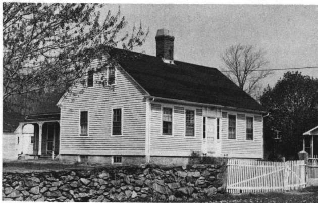
Fig. 26: Captain Esbon Sanford House (c. 1832); 88 Featherbed Lane. The farm exemplifies the transition from the Federal to the Greek Revival in rural building.
