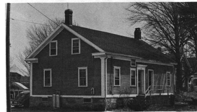
Fig. 42: I. Y. Taylor House (late 19th century); 1225 Tower Hill Road; typical late 19th-century Victorian house type built in mill villages such as Lafayette.
