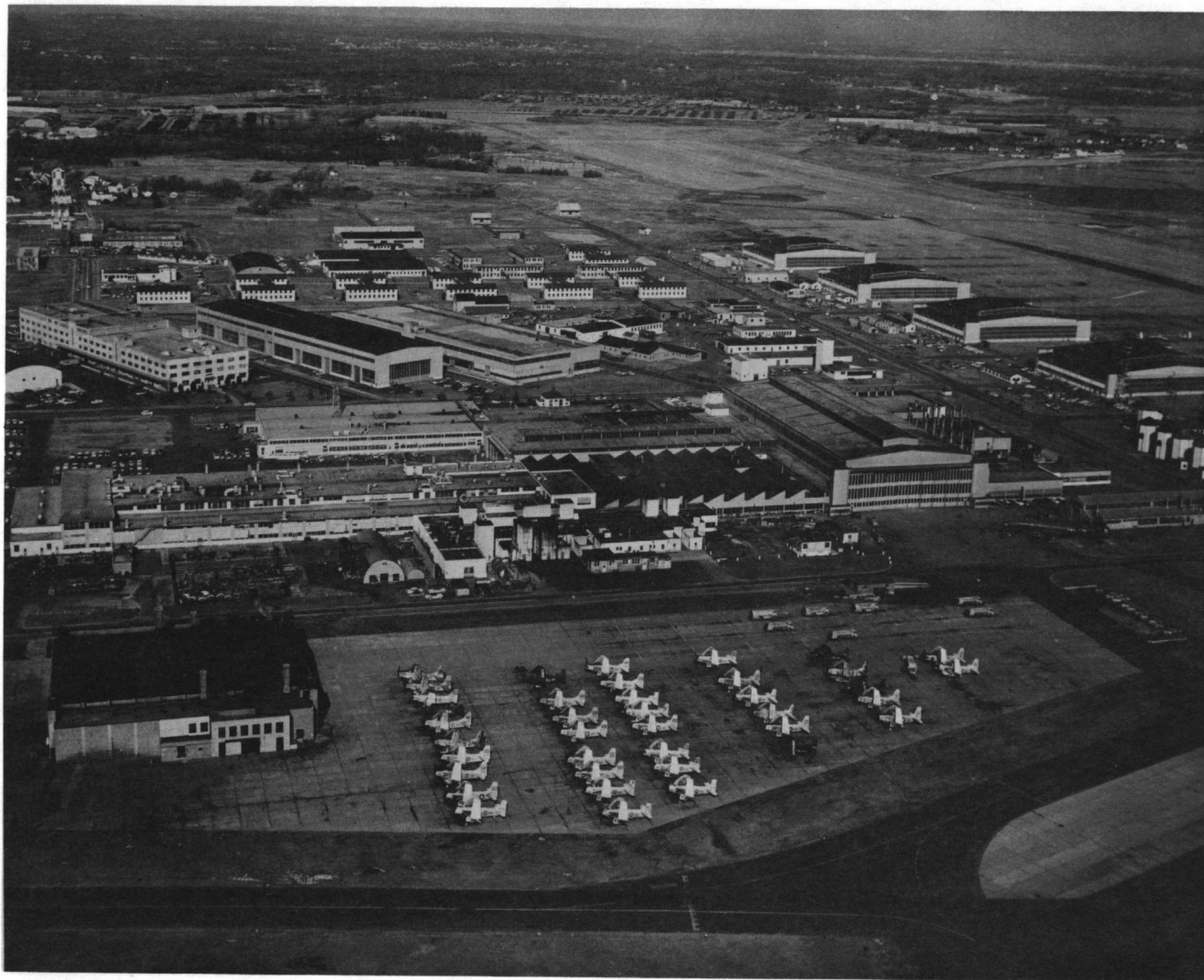
Fig. 75: Quonset Point Naval Air Station, February 12, 1958; showing Davisville in the upper left background.
