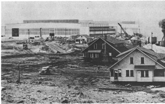
Fig. 67: Quonset Point Naval Air Station under construction; summer houses giving way to huge hangars destined to become a key war base; photograph, 1940.
