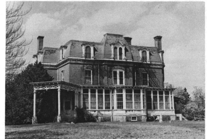
Fig. 51: Scalabrini Villa, former John Carter Brown Estate (1872); 960 North Quidnessett Road. Built in the High Victorian style with a mansard roof, Mrs. Brown gave the villa to the Rhode Island Hospital as a summer camp for crippled children; in 1957 the Society of St. Charles acquired the property for a nursing home.
