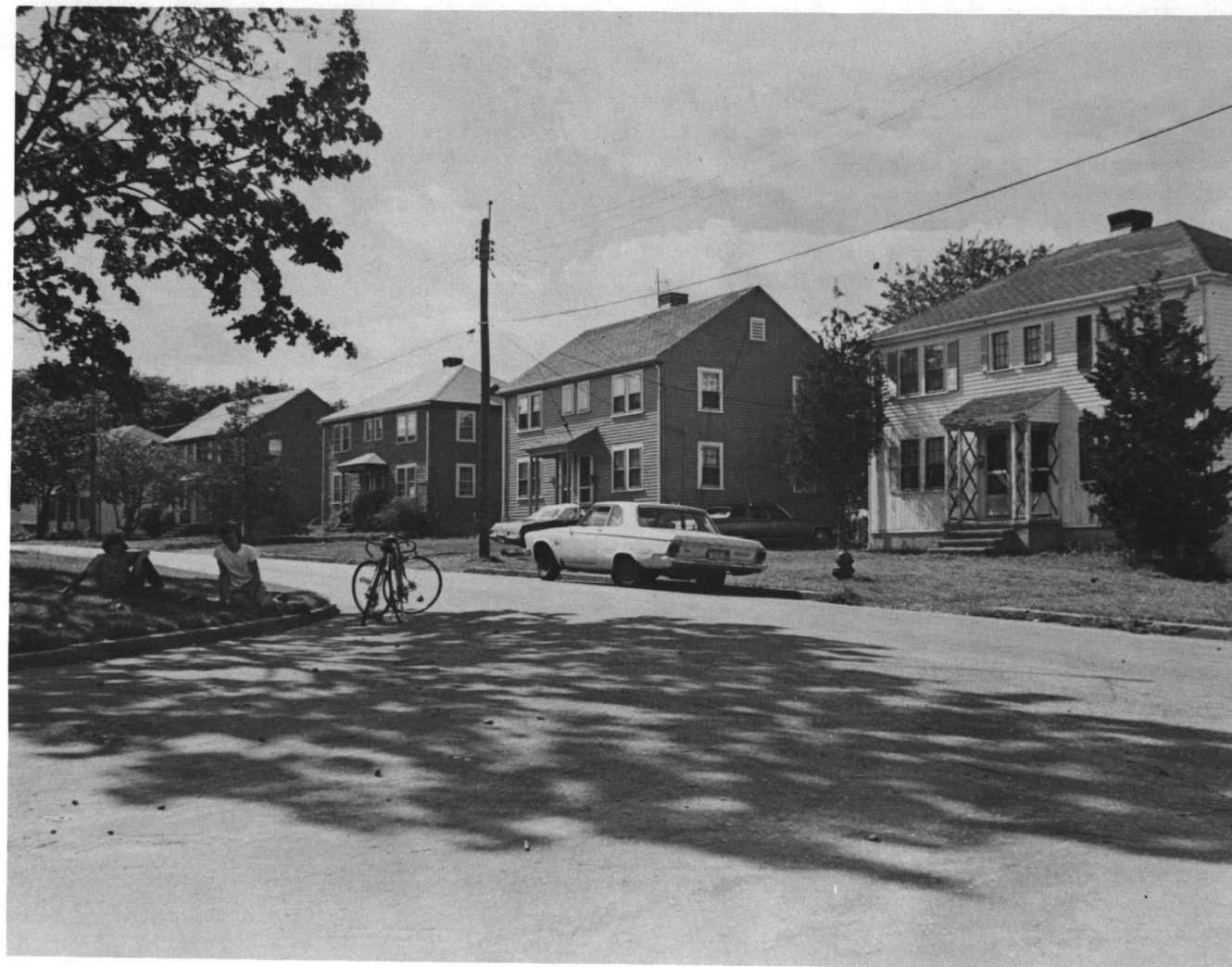
Fig. 78: Yorktown Manor (1943). This totally planned community was platted by the Massasoit Housing Corporation with Federal Housing Administration (FHA) financing; duplex homes with two entrances in the center united under a single portico, front on curving roads and share residual land between house lots reflecting advanced planning concepts of the 1930s found in "Greenbelt" villages of Maryland, Wisconsin, and Ohio.
