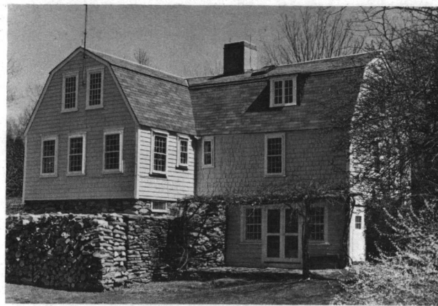
Fig. 12: Joseph Peirce House (largely 18th century with possible 17th-century parts and 19th- and 20th-century additions); 933 Gilbert Stuart Road.
