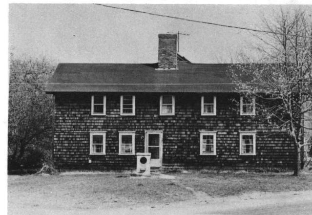
Fig. 15: Stephen Northup House (late 17th or early 18th century with mid-18th- and 19th-century additions); 99 Featherbed Lane.
