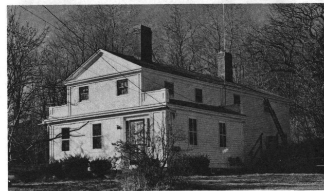
Fig. 40: Mill Supervisor's House (c. 1840); 31 Pendar Road; Silver Spring.
