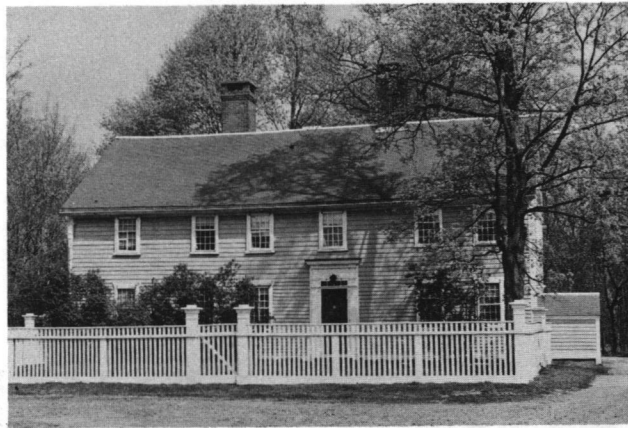
Fig. 29: Joshua Davis House (c. 1715; 1820; restored, 1948); 296 Davisville Road.
