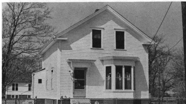
Fig. 41: Mill House (c. 1850s); 1310 Tower Hill Road; typical of the Greek Revival type double house built for workers at the nearby Shady Lea or Silver Spring mills.
