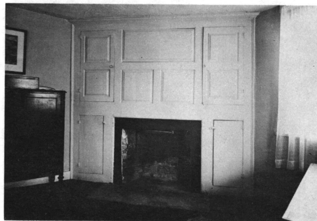
Fig. 14: Interior, Hall-Northup House (1638?; c. 1676; enlarged, c. 1745); shows typical 18th-century paneling; 7919 Post Road.
