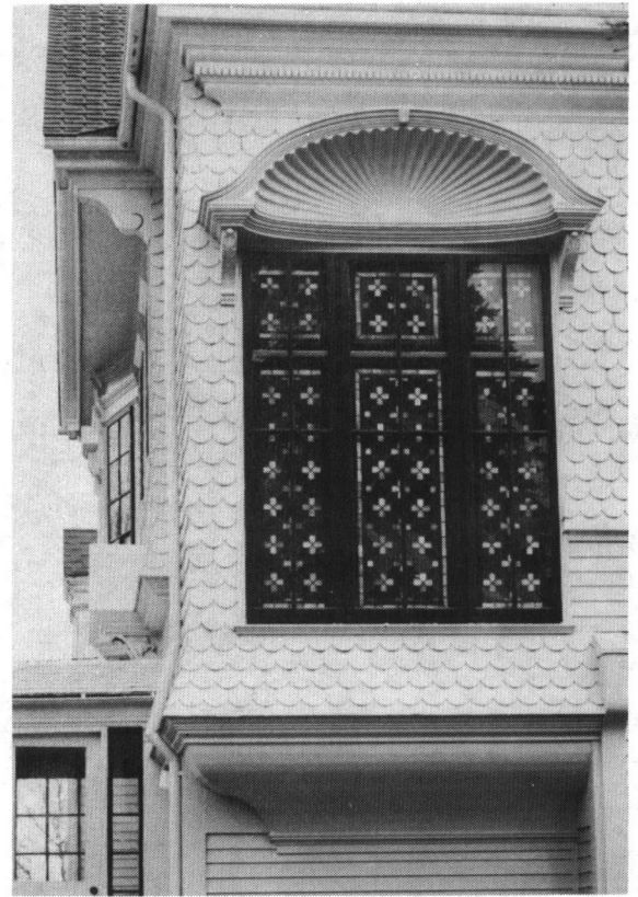
F. 34 THE MORRIS HOUSE (1882-83) 86 RHODE ISLAND AVENUE
