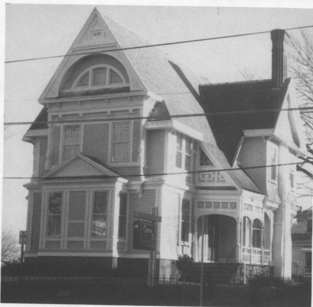
Town Hall (1894); 45 Broad Street
