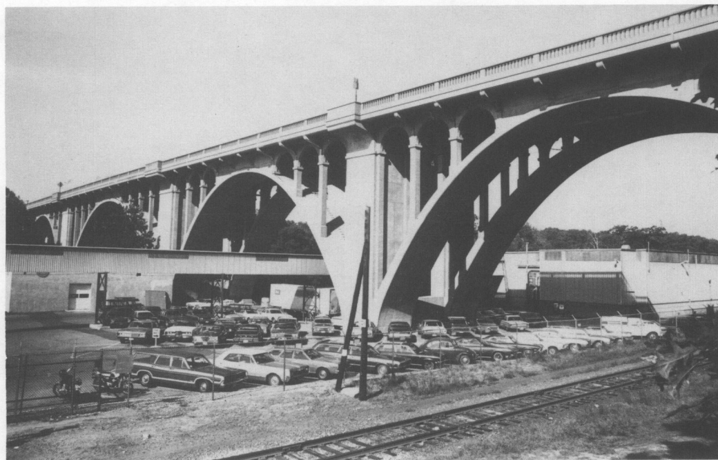
Ashon Viaduct (1934-45); George Washington Highway
