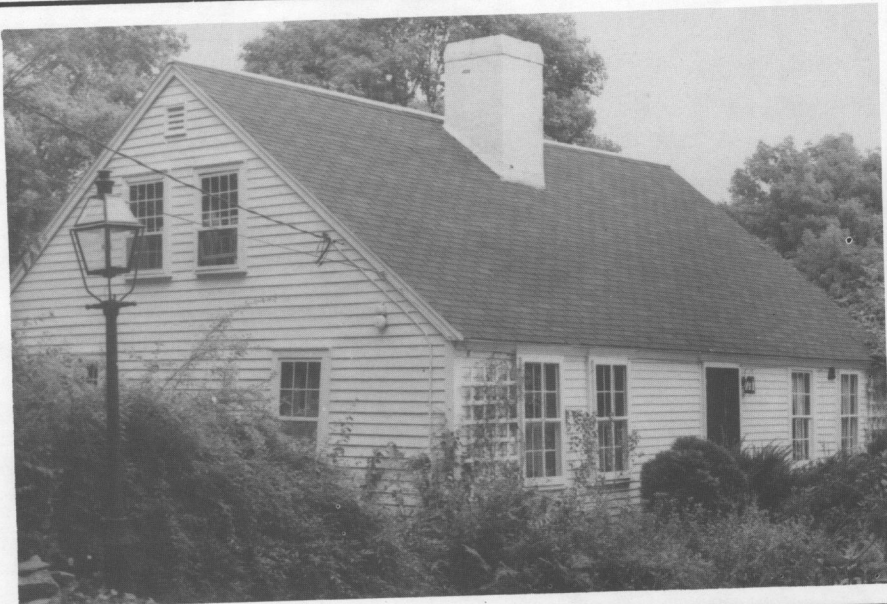
Hixon Homestead/Maple Shade Farm (late 17th century); 27 Hines Road
