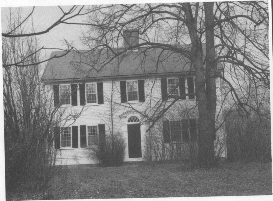
Miller House (c. 1797); Tower Hill Road
