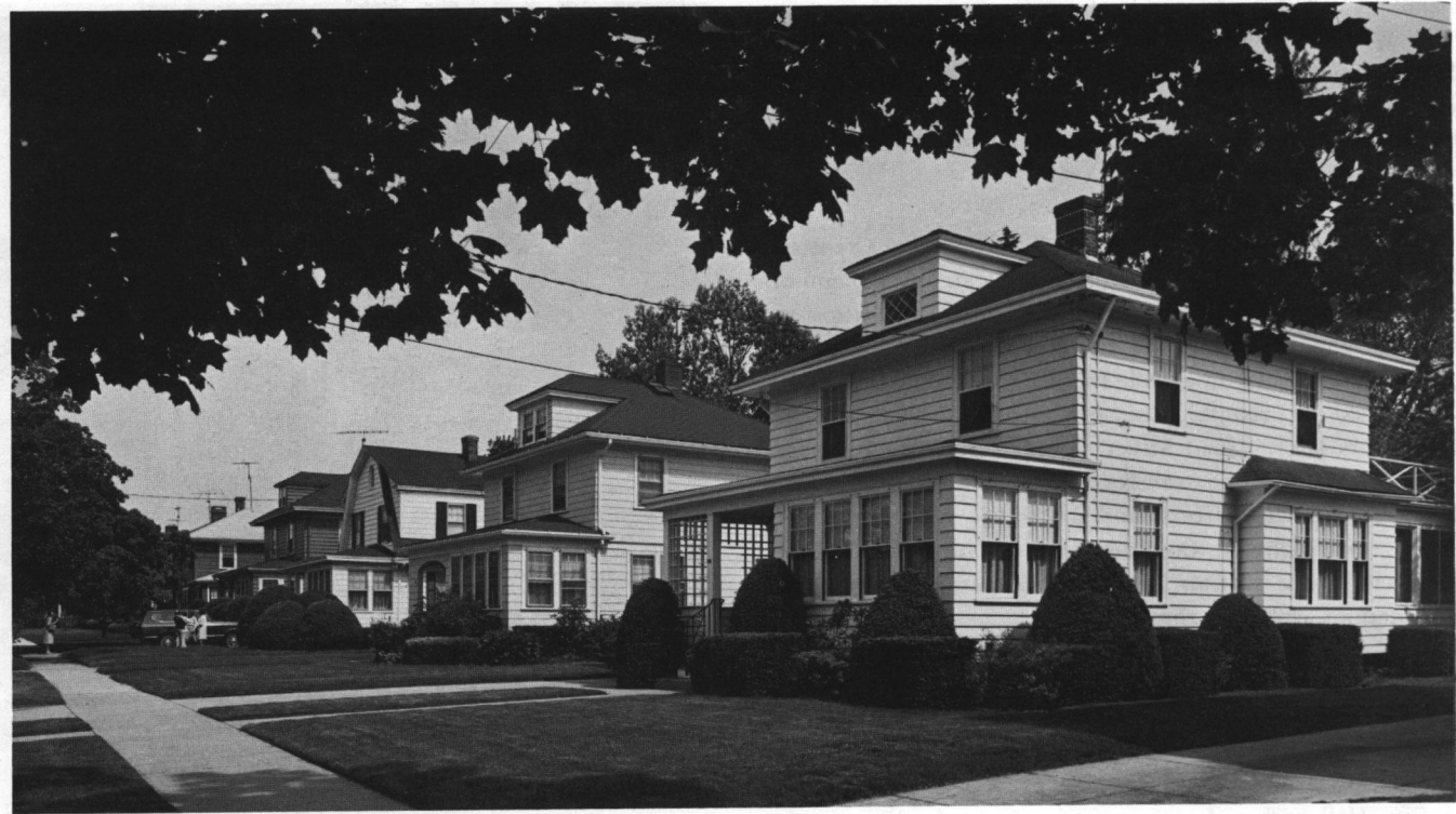
Fig. 73: Twentieth-century houses along Shirley Boulevard; Auburn.
