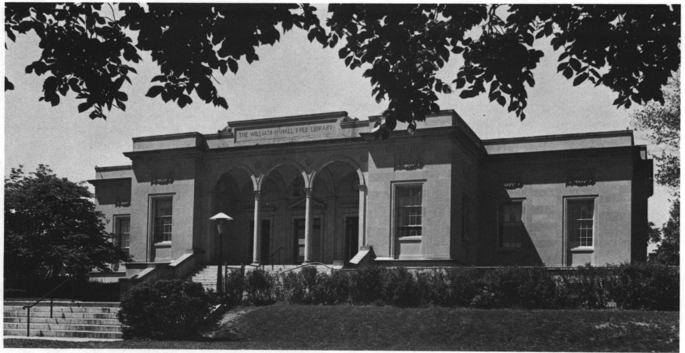
Fig. 70: William H. Hall Free Library (1927); 1825 Broad Street; architect, George Martin Hall.
