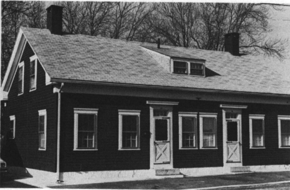
Fig. 10: 38-40 Oak Street (c. 1864): A late Greek Revival, two-family mill house built by the Cranston Print Works.
