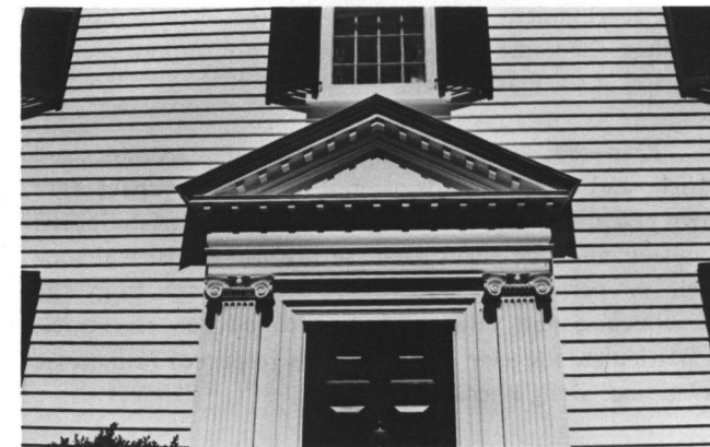
Fig. 7: 1231 Hope Road (c. 1790): A fine Late Georgian doorway with Ionic pilasters; compare with Fig. 6.
