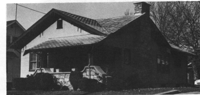
Fig. 26: 77 Edgewood Avenue (c. 1927): A bungalow with characteristic intersecting roof planes and recessed porch.
