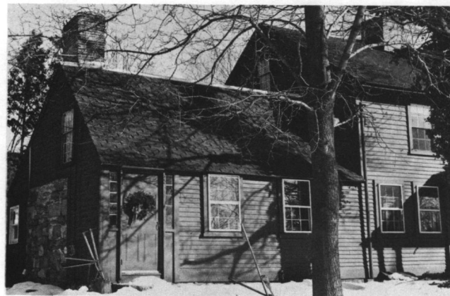
Fig. 11: Edward Searle House (1677); 109 Wilbur Avenue. Two-story portion added to "stone-ender" by 1727.
