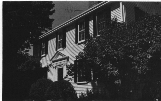
Fig. 3: 1231 Hope Road (1735, 1790): The classic, center-chimney, gable-roofed, central-entrance, 4-bay facade, 18th-century house. The type persisted for a century.
