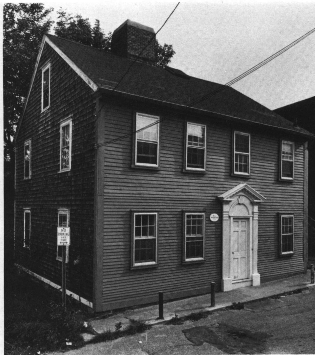
Fig. 13: Remington Arnold House (c. 1730); 12 Bridge Street, Pawtuxet.
