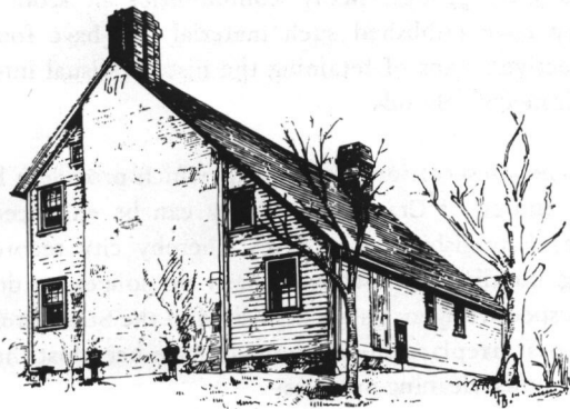
Fig. 1: 1580 Plainfield Pike (c. 1677): A late seventeenth-century 2-story, “stone-ender,” built on a one-room ground plan.
