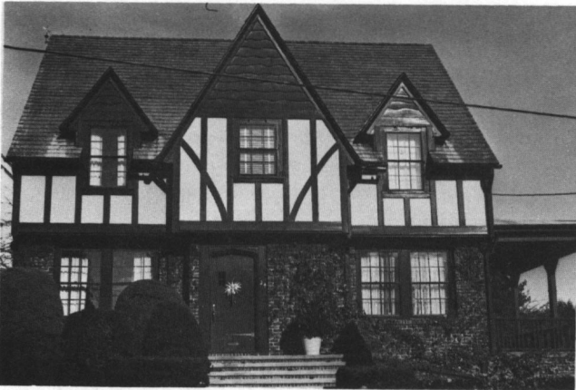
Fig. 28: 24 Harbour Terrace (c. 1938): A pseudo-Tudor house with "garrison" overhang and half-timbering.
