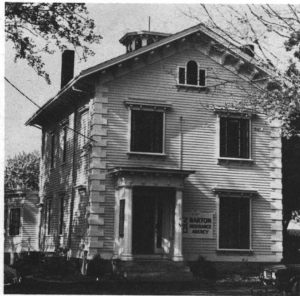
Fig. 12: 407 Pontiac Avenue (c. 1858): The same basic house as Fig. 11, but with Bracketed Style detail and corner quoins.
