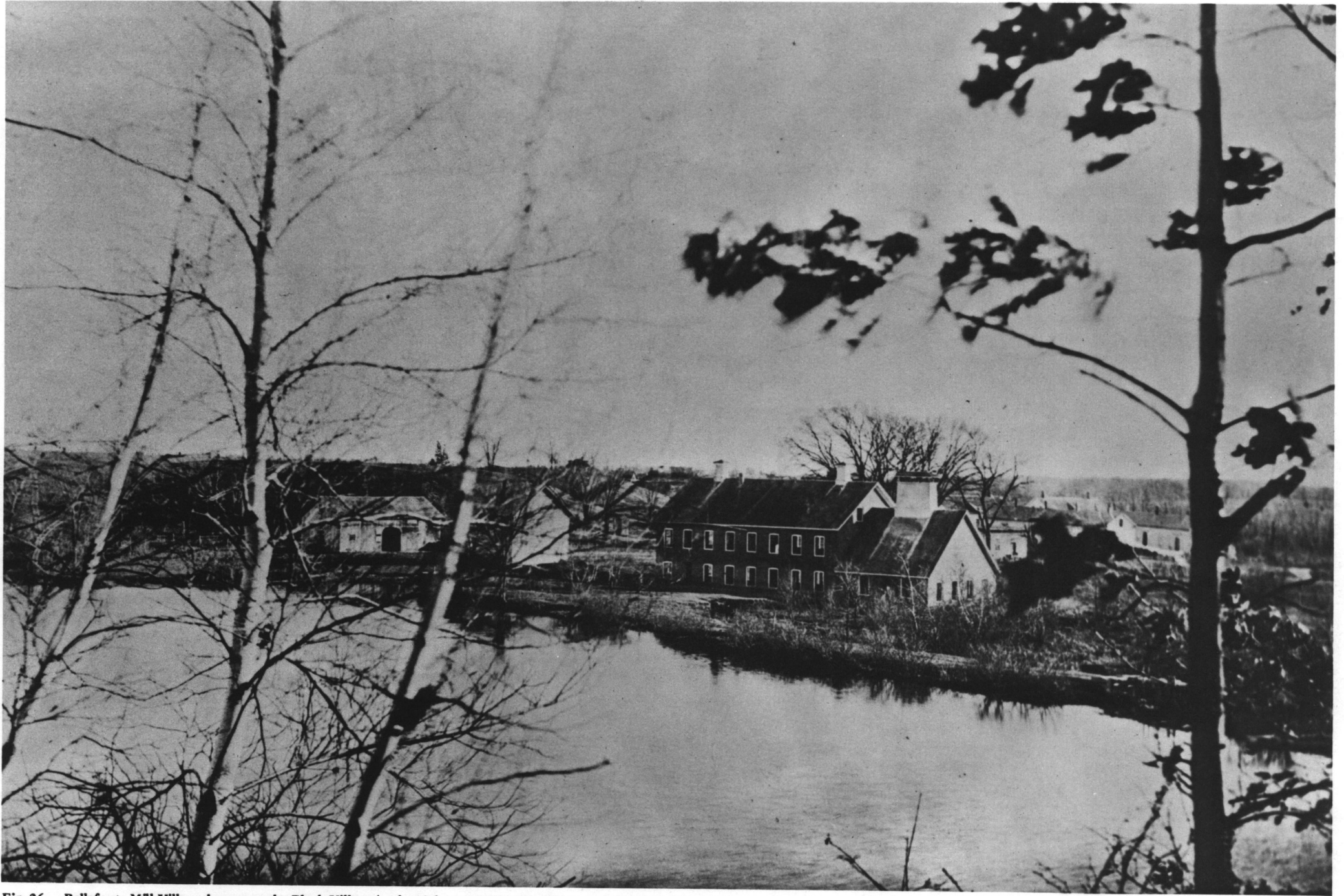
Fig. 26: Bellefonte Mill Village, known as the Black Village (early 19th century); originally part of the C. and W. Rhodes textile empire, much of the complex was burned in 1870. It was acquired the following year by the Turkey Red Dye Company. In 1911 the Imperial Printing and Finishing Company was established here.
