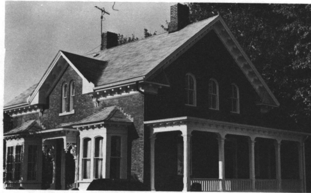
Fig. 13: 12 Talbot Manor (c. 1864): An elaborate Bracketed cottage with a cross gable, bay windows and entrance hood.
