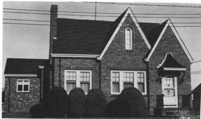
Fig. 29: 35 Calaman Road (c. 1934): An early 20th-century "English Cottage" with heavy, steep gables.
