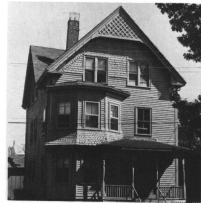
Fig. 17: 15-17 Bain Street (c. 1900): The same house as Figs. 15 and 16, but with Queen Anne trim.
