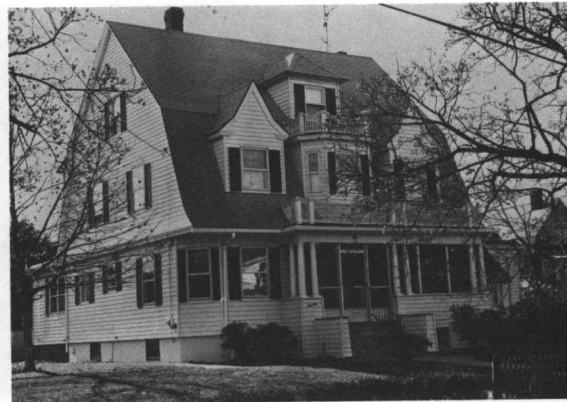
Fig. 22: 14 Glen Avenue (1904): A typical, Queen Anne-Colonial Revival with complex gambrel roof and multiple dormers.
