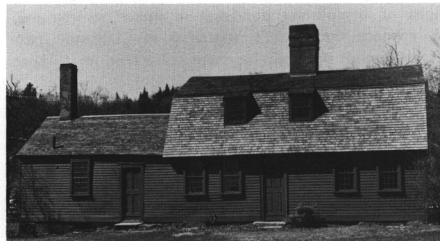
Fig. 5: 156 Scituate Avenue (c. 1764): A common, Cranston 18th-century hometype; one-and-one-half-story, gambrel-roofed, 5-bay facade, center-chimney dwelling.
