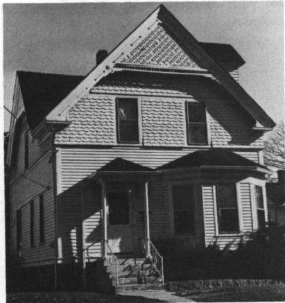
Fig. 19: 240 Pawtuxet Avenue (c. 1890): A typical Queen Anne cottage with patterned shingling and bargeboard.
