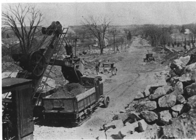
Fig. 72: Road construction on Natick Avenue; photograph, c. 1903.
