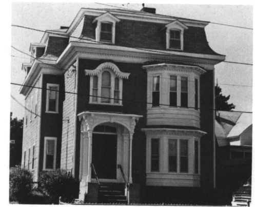
Fig. 15: 24-26 Whipple Avenue (c. 1875): A typically urban house with mansard roof, side-hall entry and 2-story bay window.
