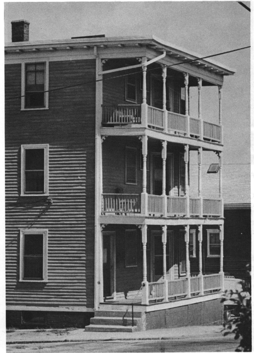
Figure 45: House, c. 1890; 59-61 Cross Street.
