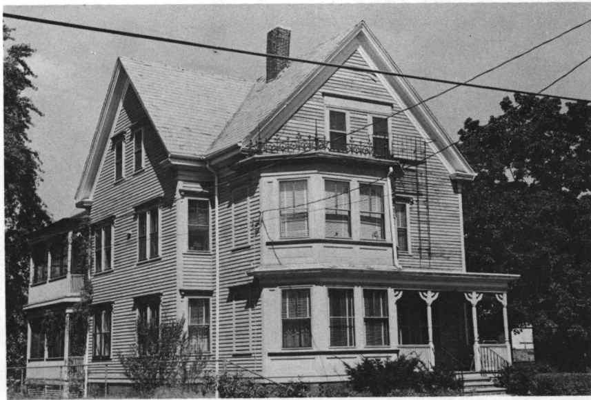
Figure 44: House, 1880s; 311-313 Central Street.
