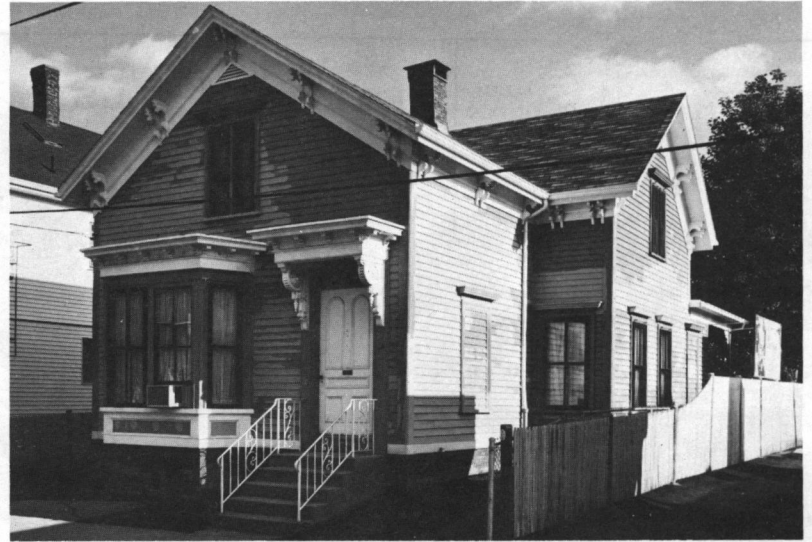
Figure 36: Horton House, 1850s; 78 Jenks Street.
