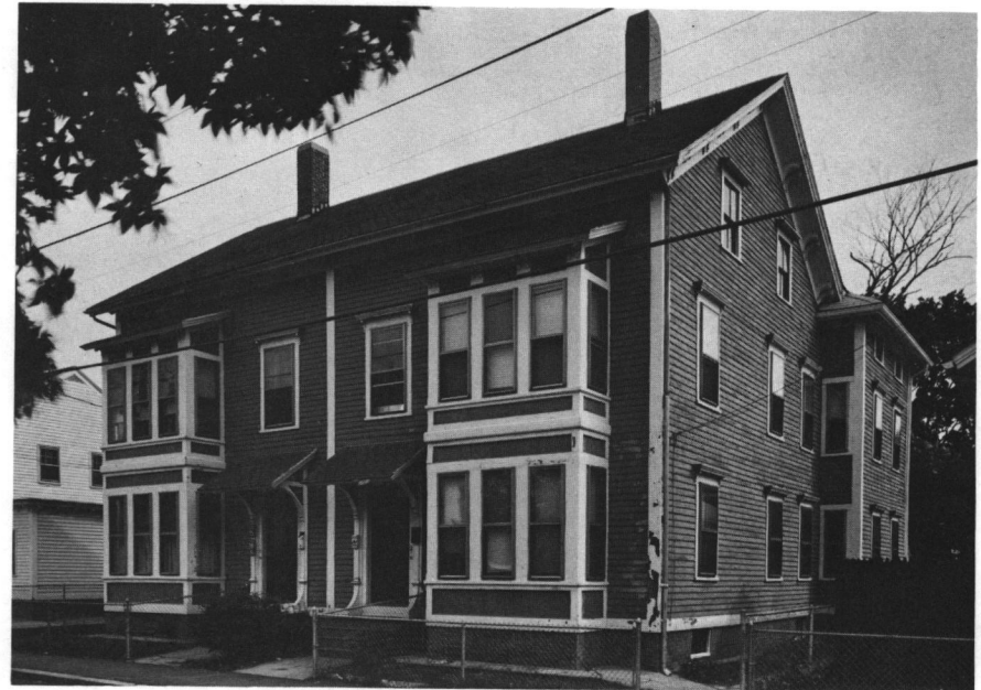
Figure 43: House, 1880s; 234-236 Central Street.
