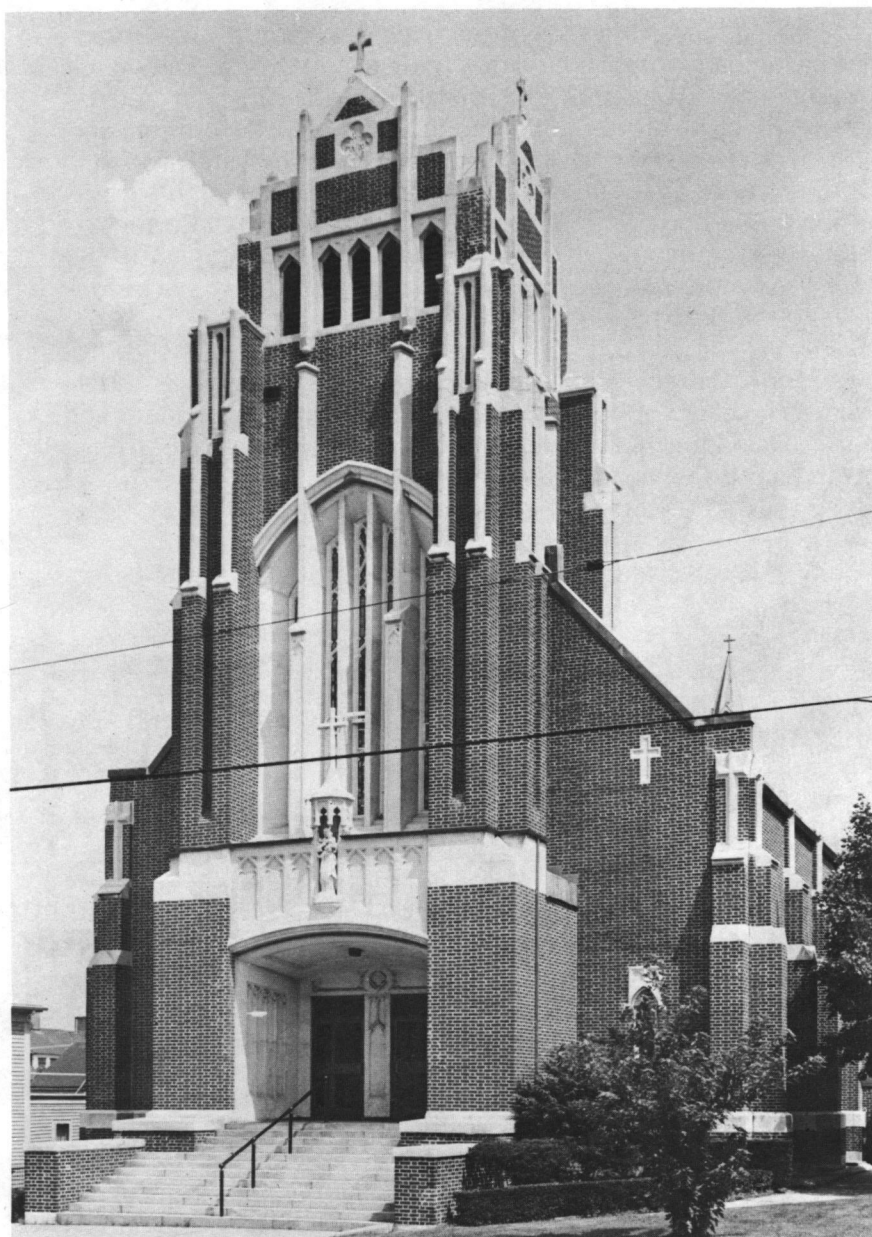
Figure 50: Church of St. Joseph, 1919; 391 High Street.
