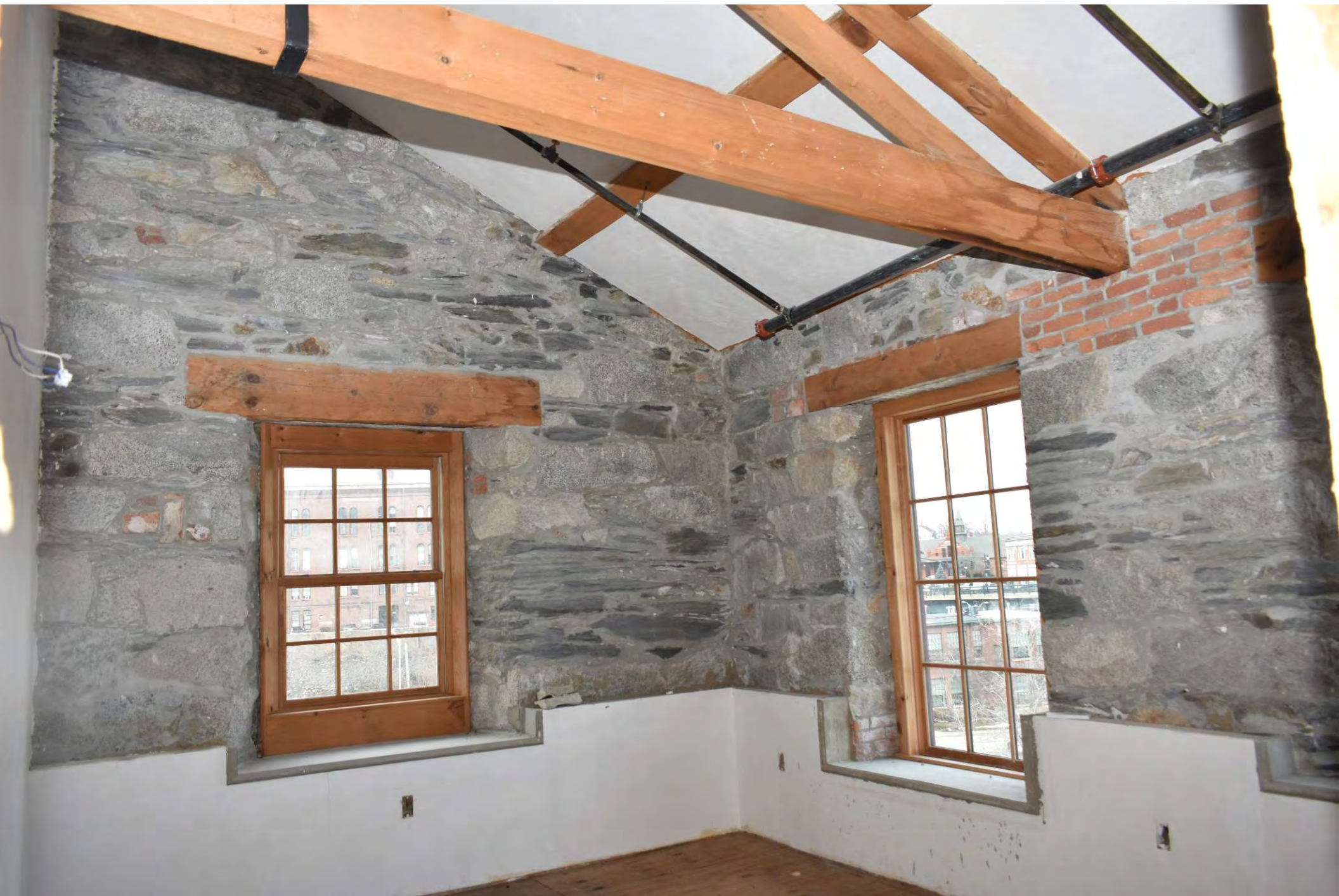
Photo 15 of 30: #2 Mill fourth floor, facing northwest
