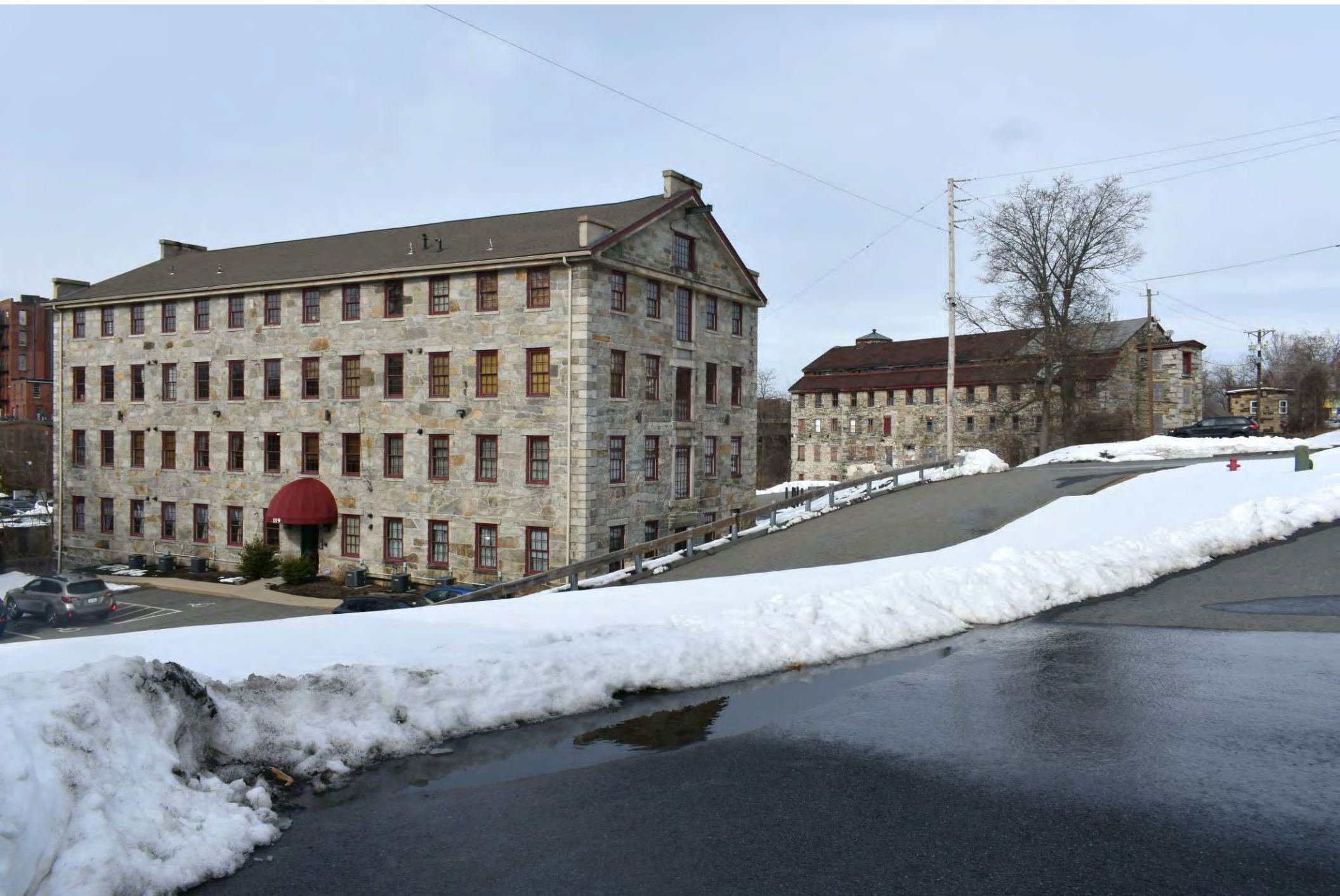
Photo 13 of 30: #2 Mill (left) and #1 Mill (right), south and east elevations, facing northwest
