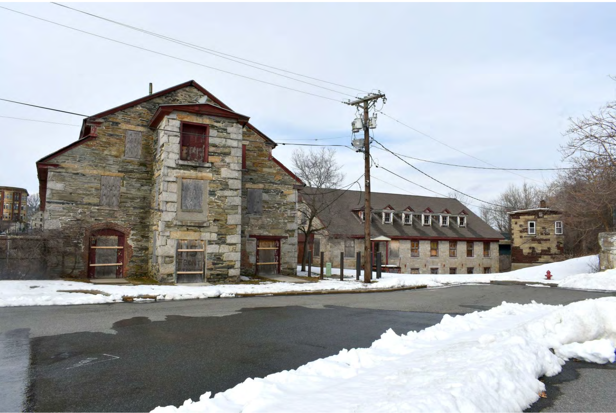
Photo 1 of 30: # 1 Mill (left) and #4 Mill (right), east elevations, facing northwest
