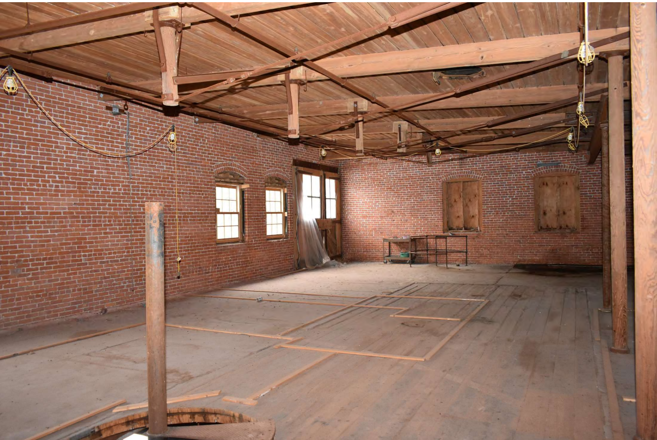
Photo 23 of 30: Garage, second floor, facing northeast
