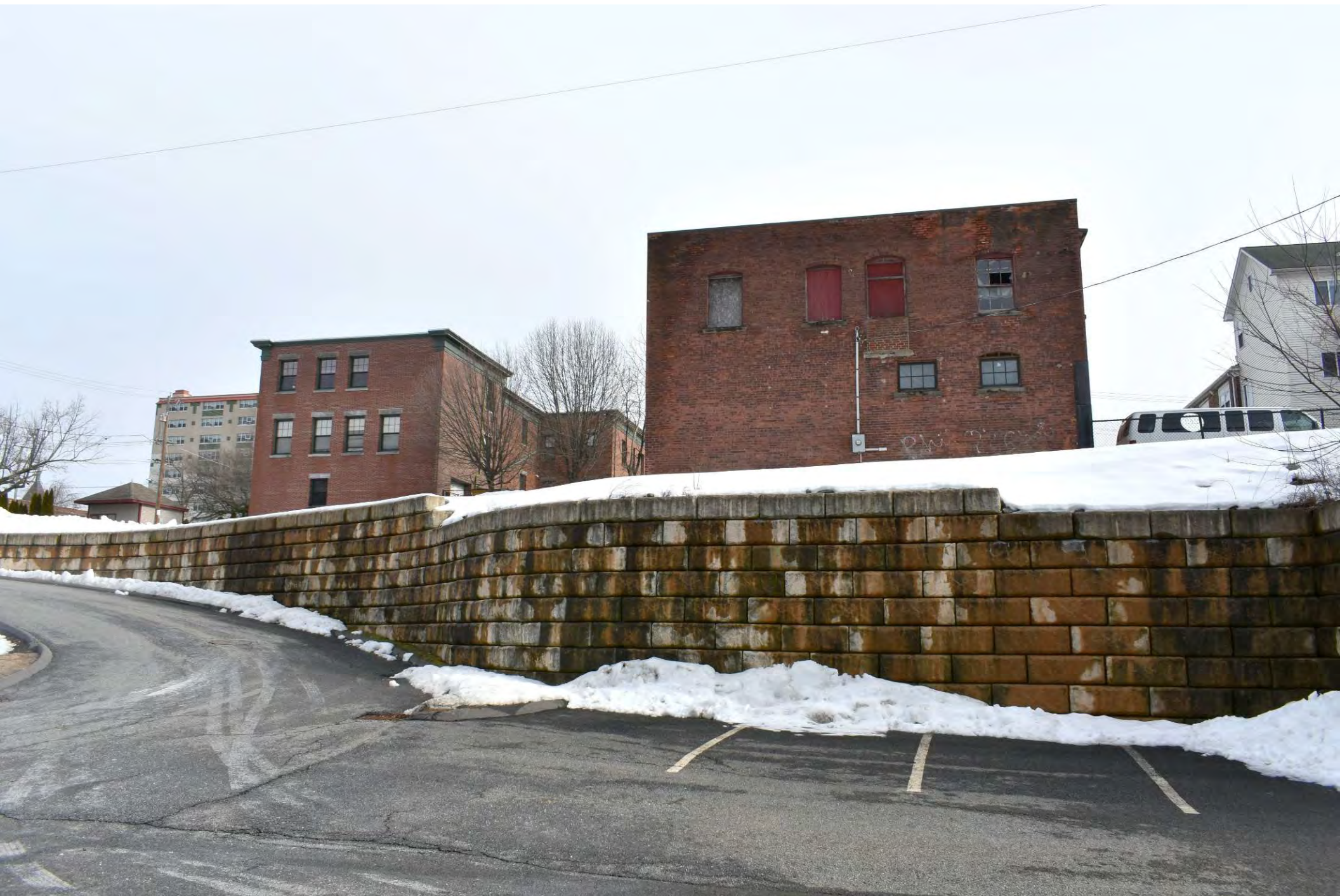
Photo 20 of 30: Garage, west elevation, facing east
