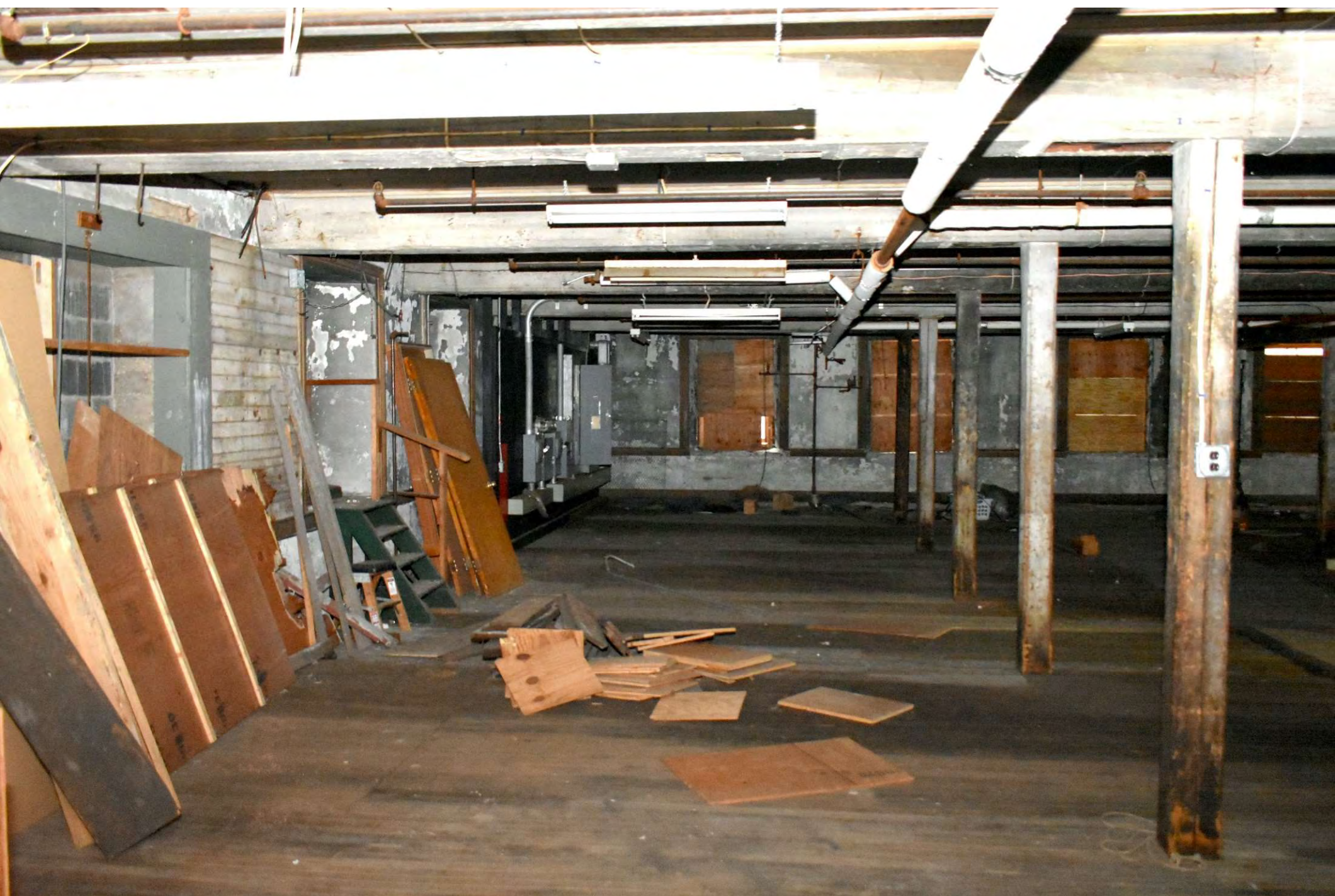
Photo 10 of 30: #4 Mill, second floor, facing north
