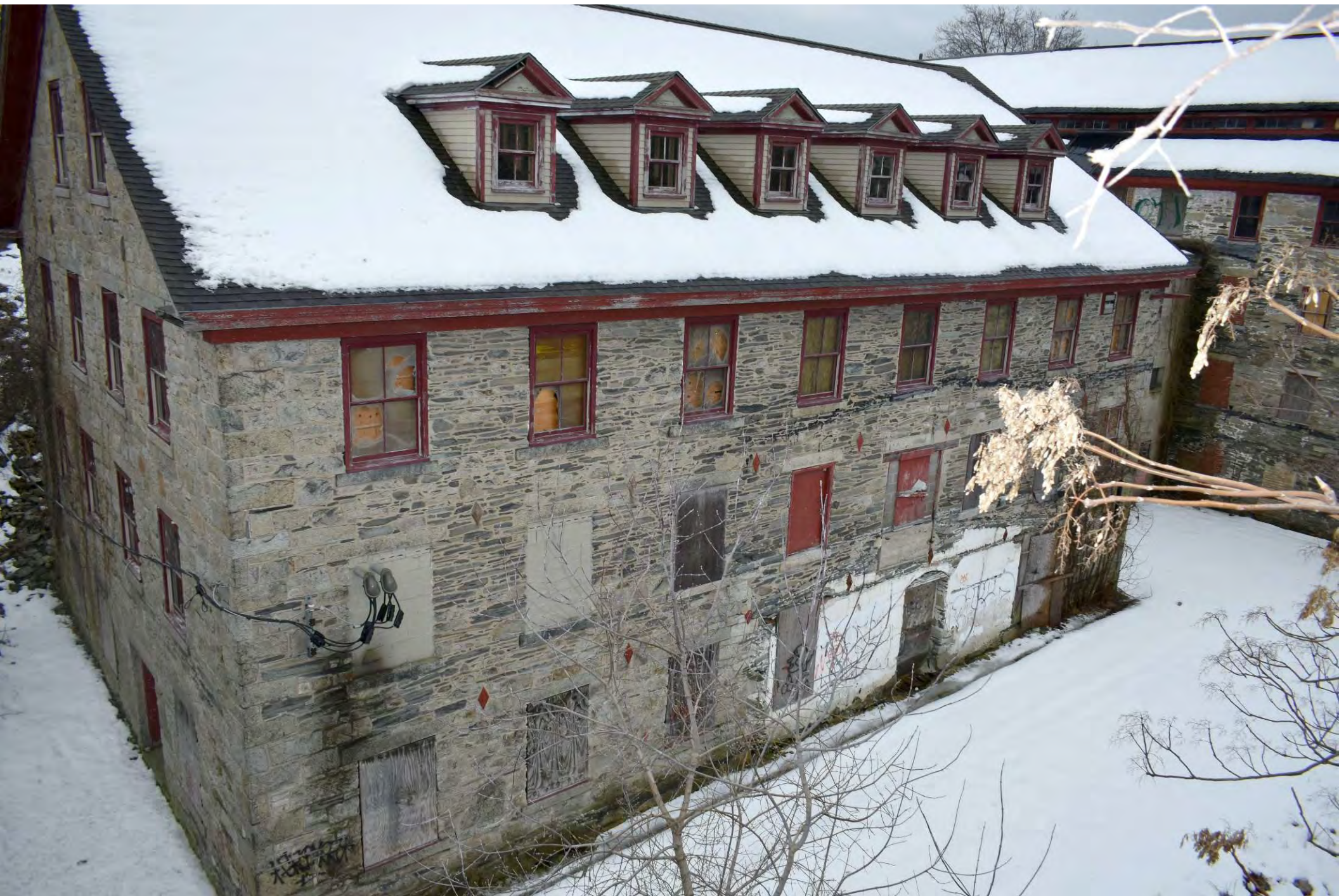
Photo 9 of 30: #4 Mill, north and west elevations, facing southeast
