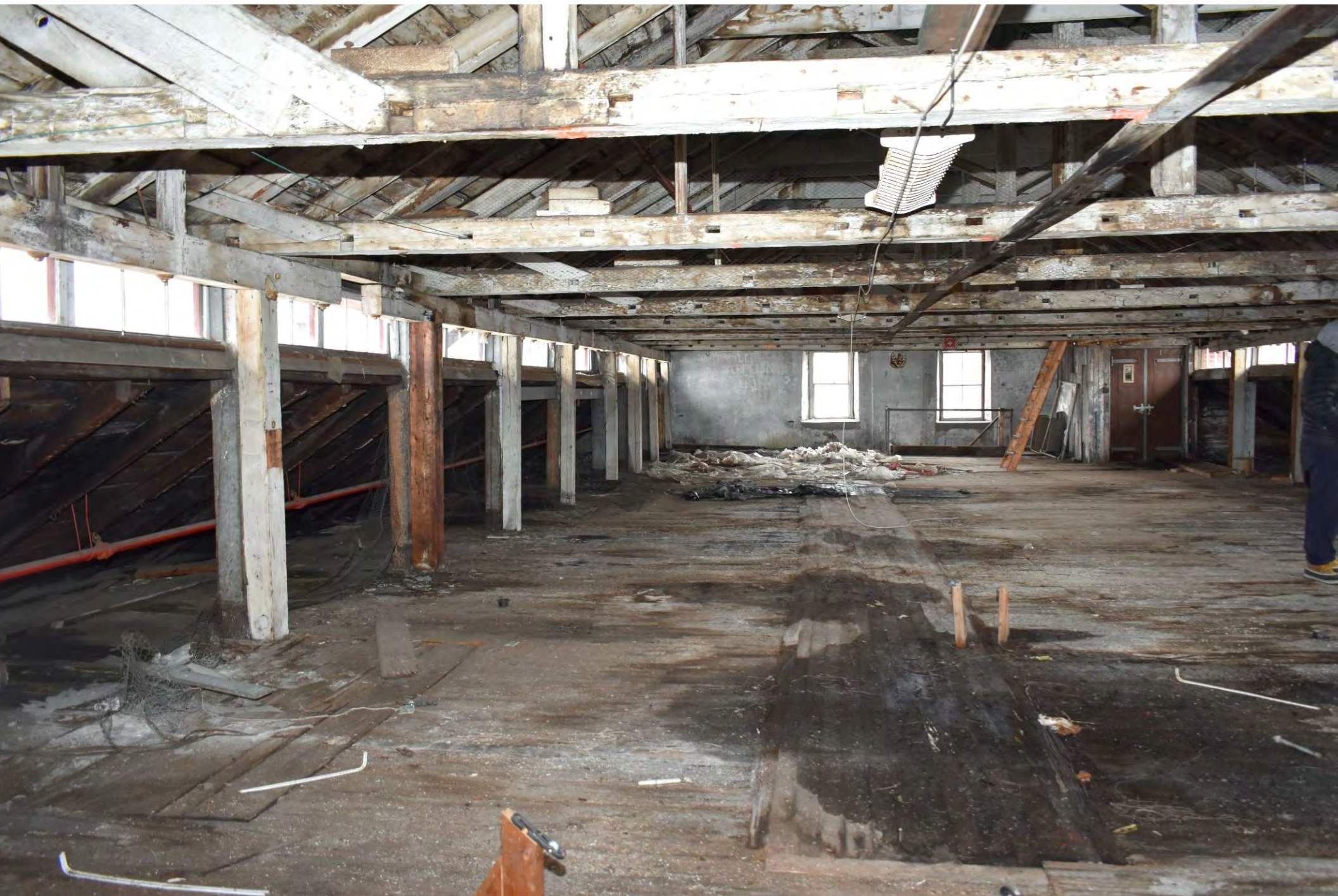
Photo 7 of 30: # 1 Mill, attic, facing west
