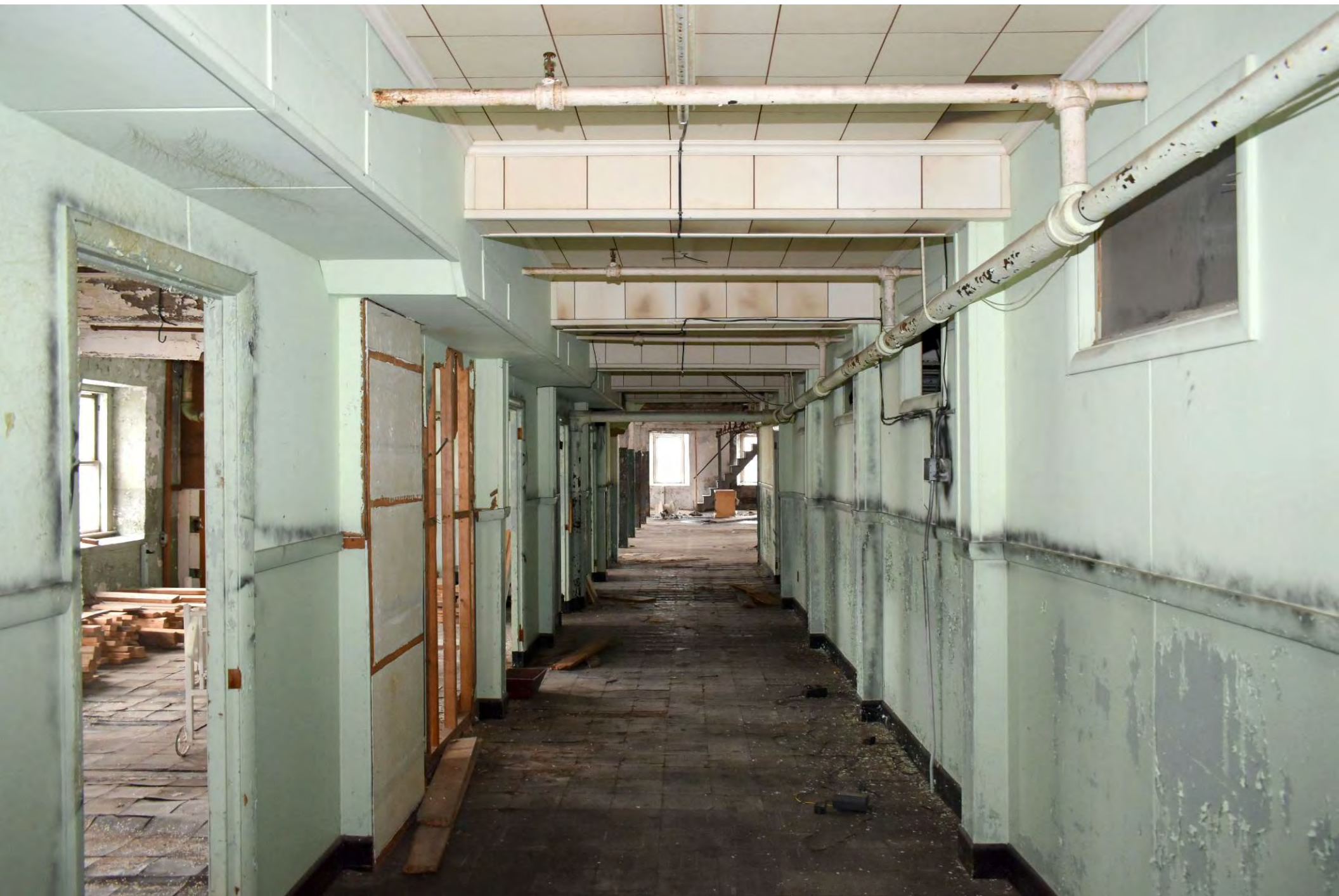
Photo 6 of 30: # 1 Mill, third floor, facing west
