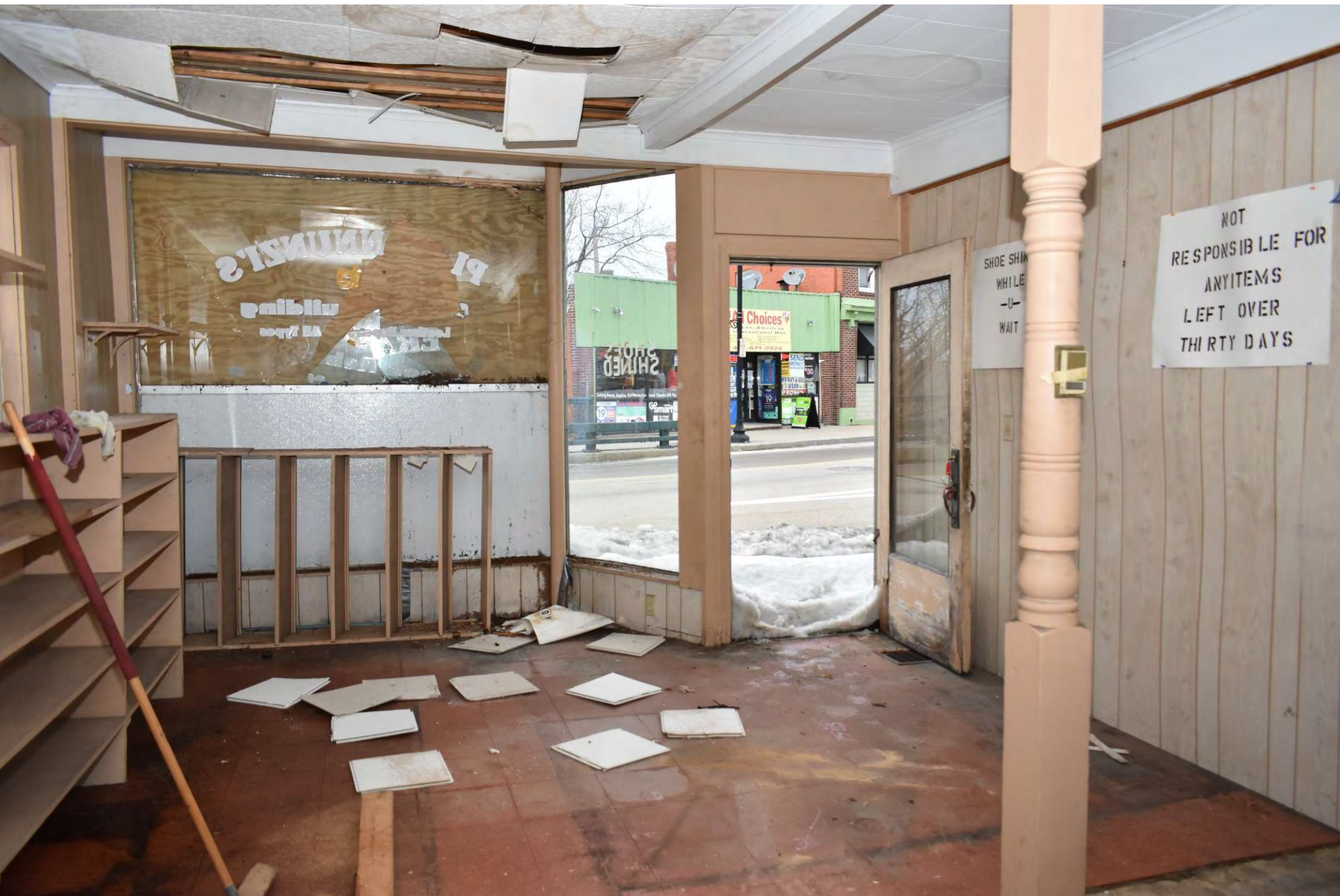
Photo 28 of 30: 125 Court Street, first floor, facing north
