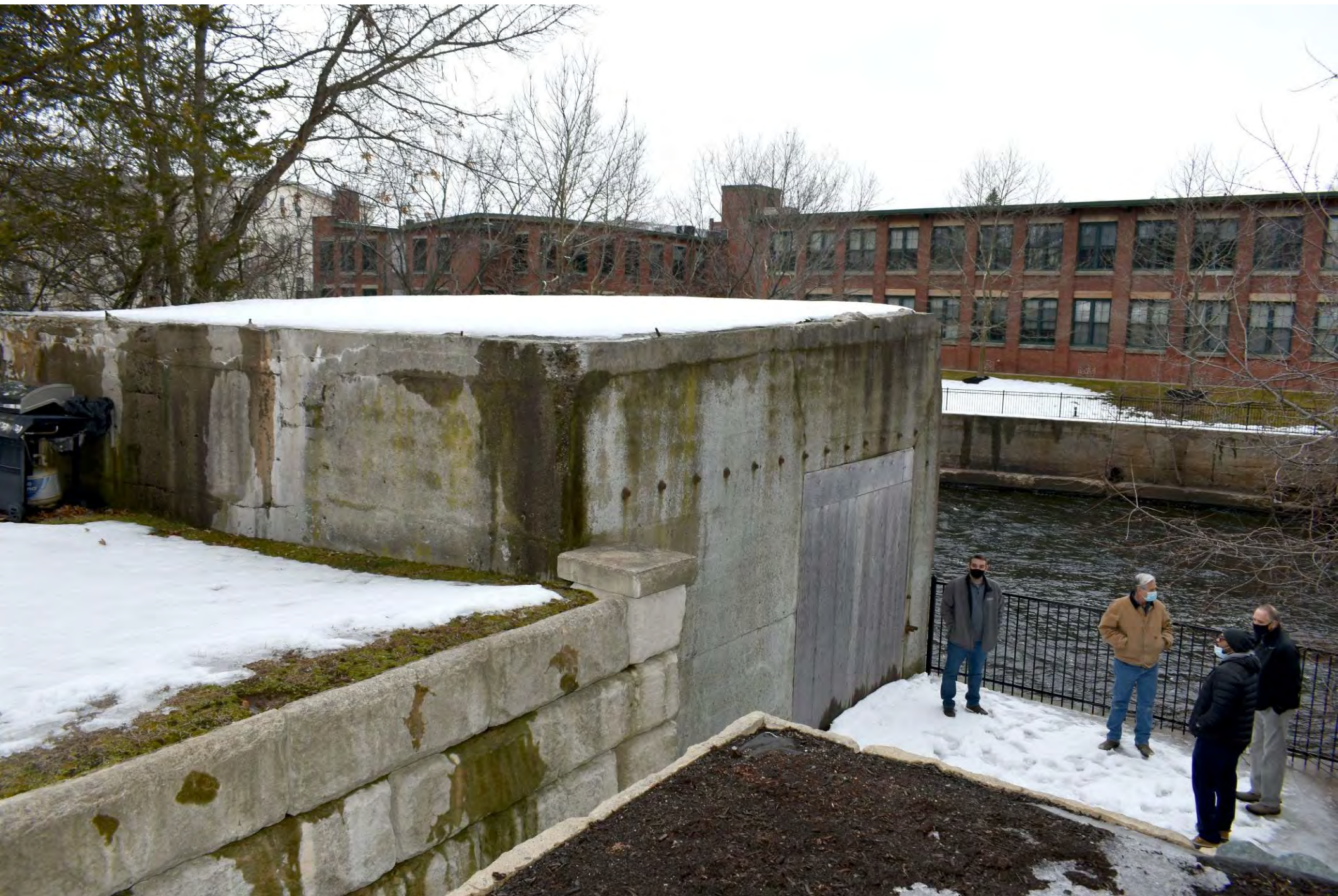
Photo 18 of 30: Power House, east and north elevations, facing southwest
