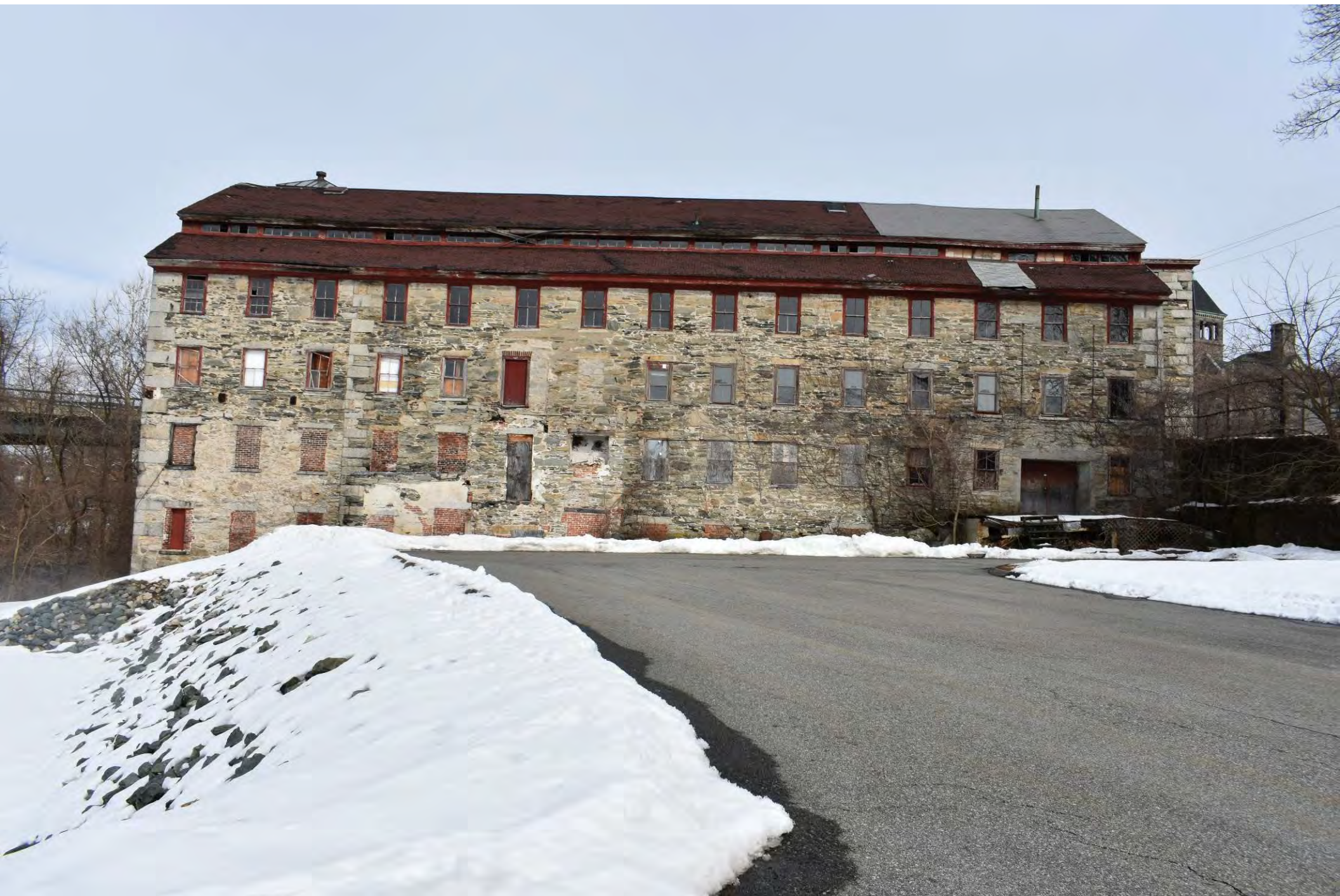
Photo 3 of 30: # 1 Mill, south elevation, facing northeast
