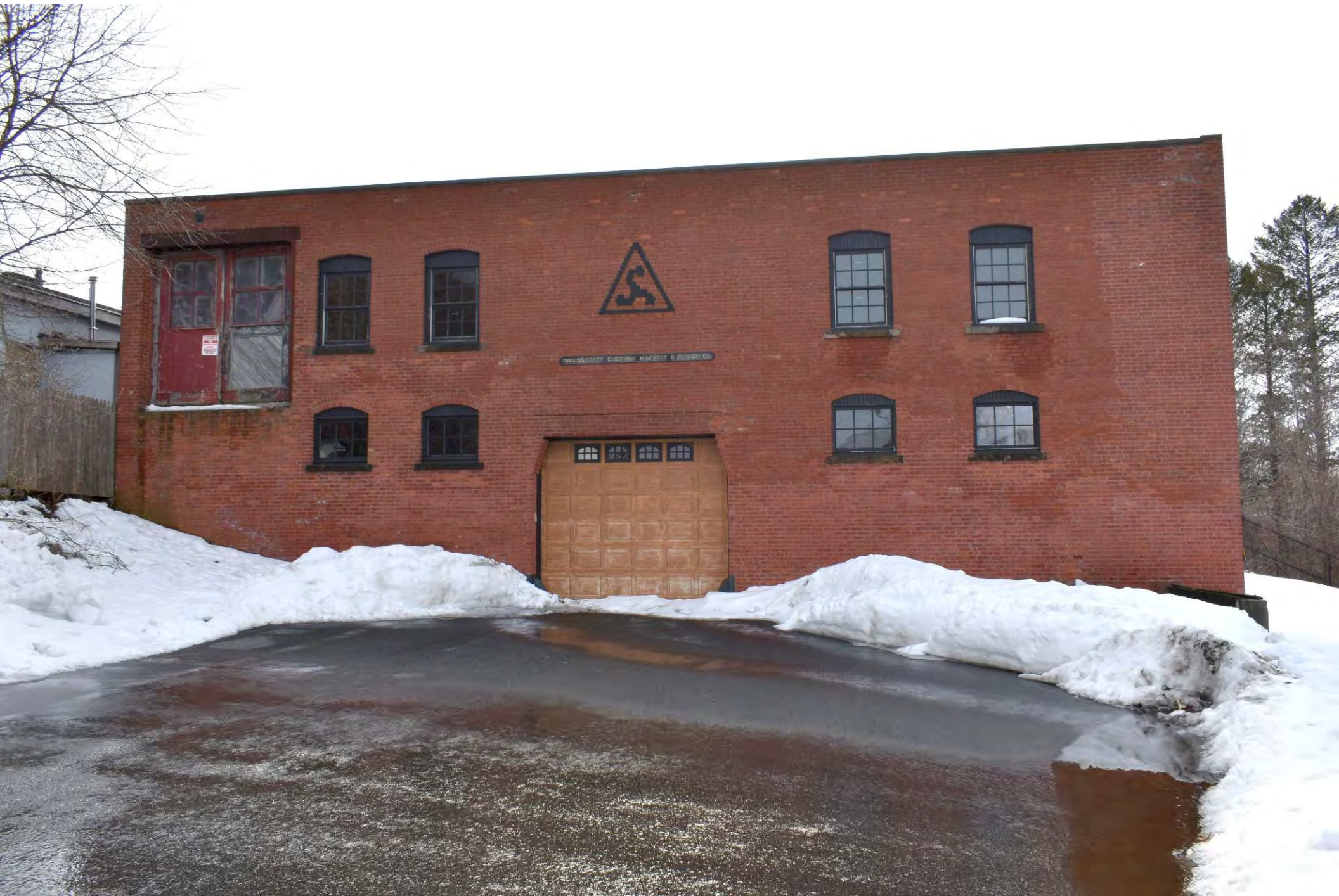
Photo 19 of 30: Garage, north elevation, facing south
