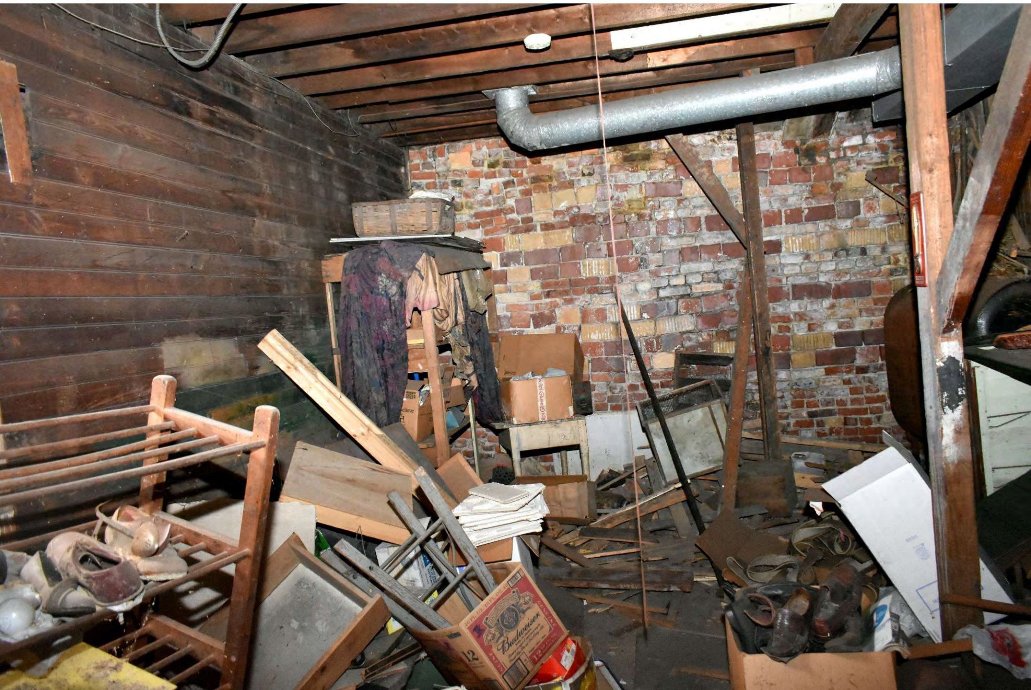
Photo 27 of 30: 125 Court Street, basement, facing south
