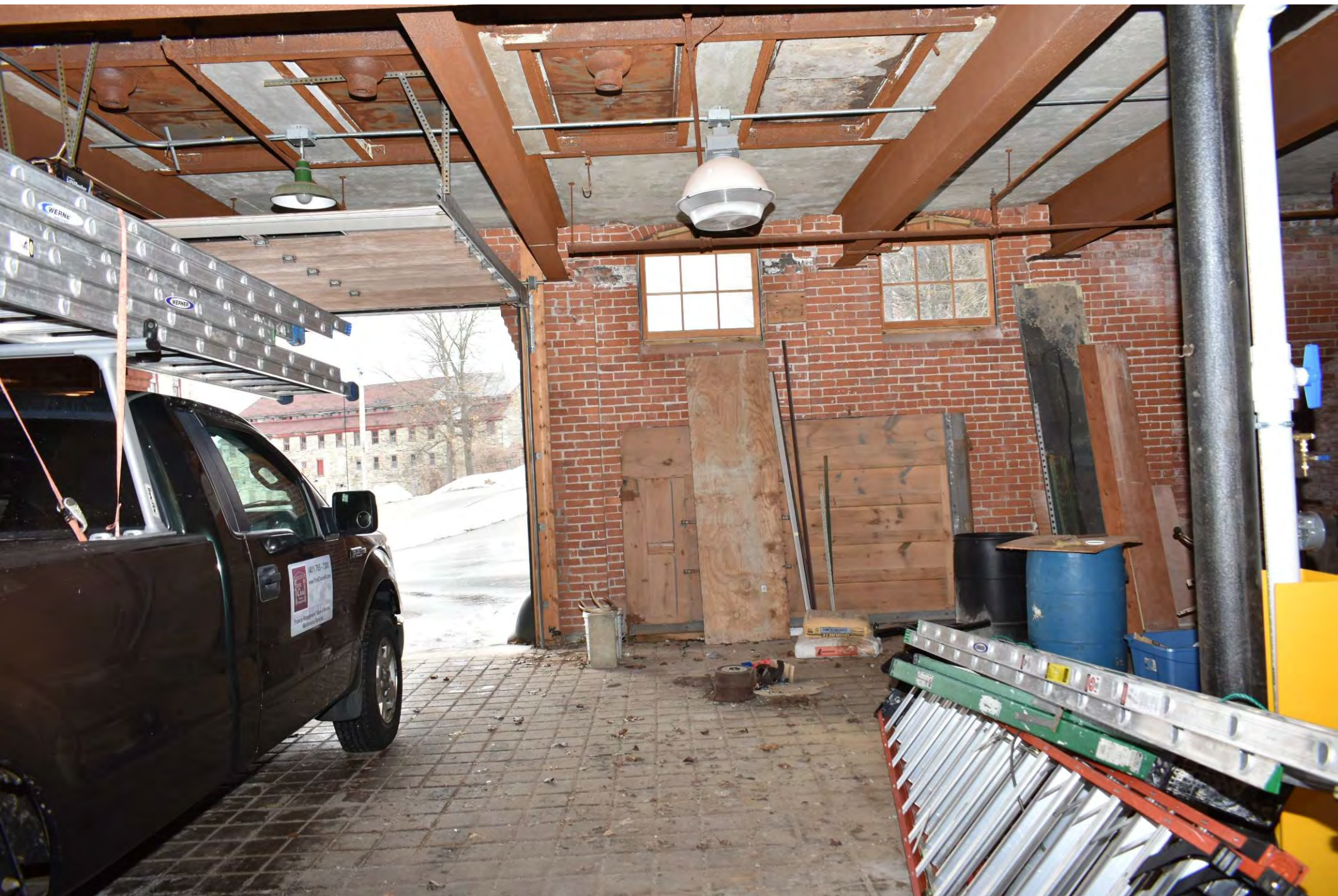
Photo 22 of 30: Garage, first floor, facing north
