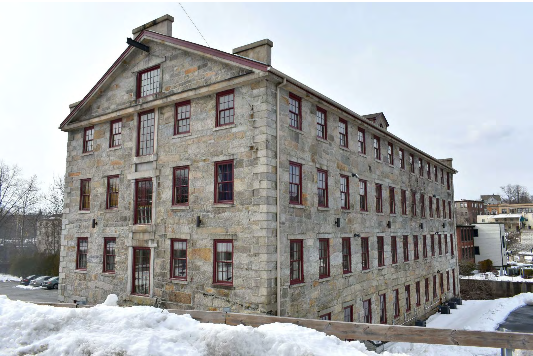
Photo 12 of 30: #2 Mill east and north elevations, facing southwest
