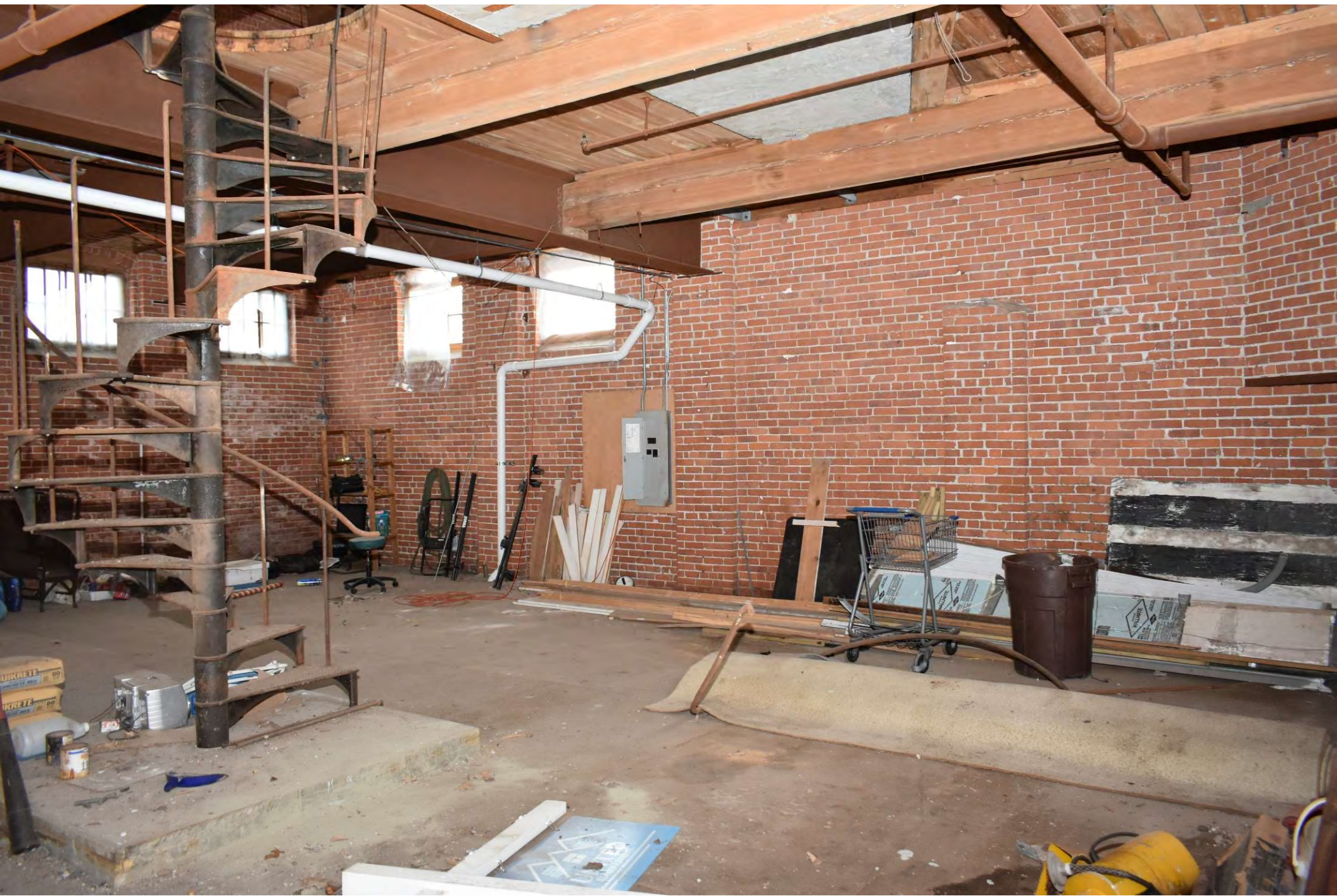
Photo 21 of 30: Garage, first floor, facing southwest
