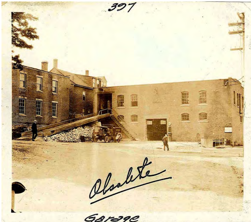
Figure 2: Early-20 th century photo showing the Garage's north and west elevations. Source: private collection of Jeffrey Emidy.
