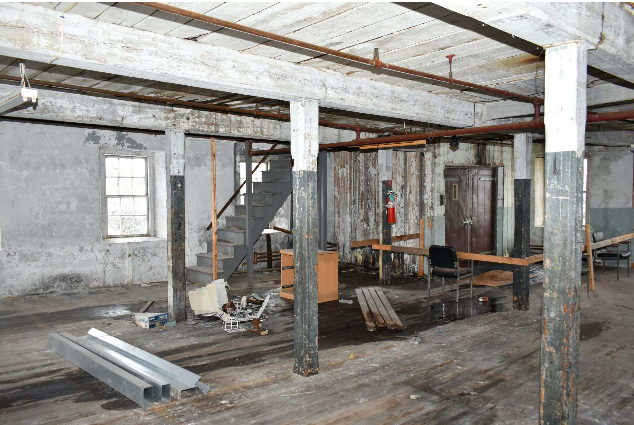
Photo 5 of 30: # 1 Mill, third floor, facing northwest
