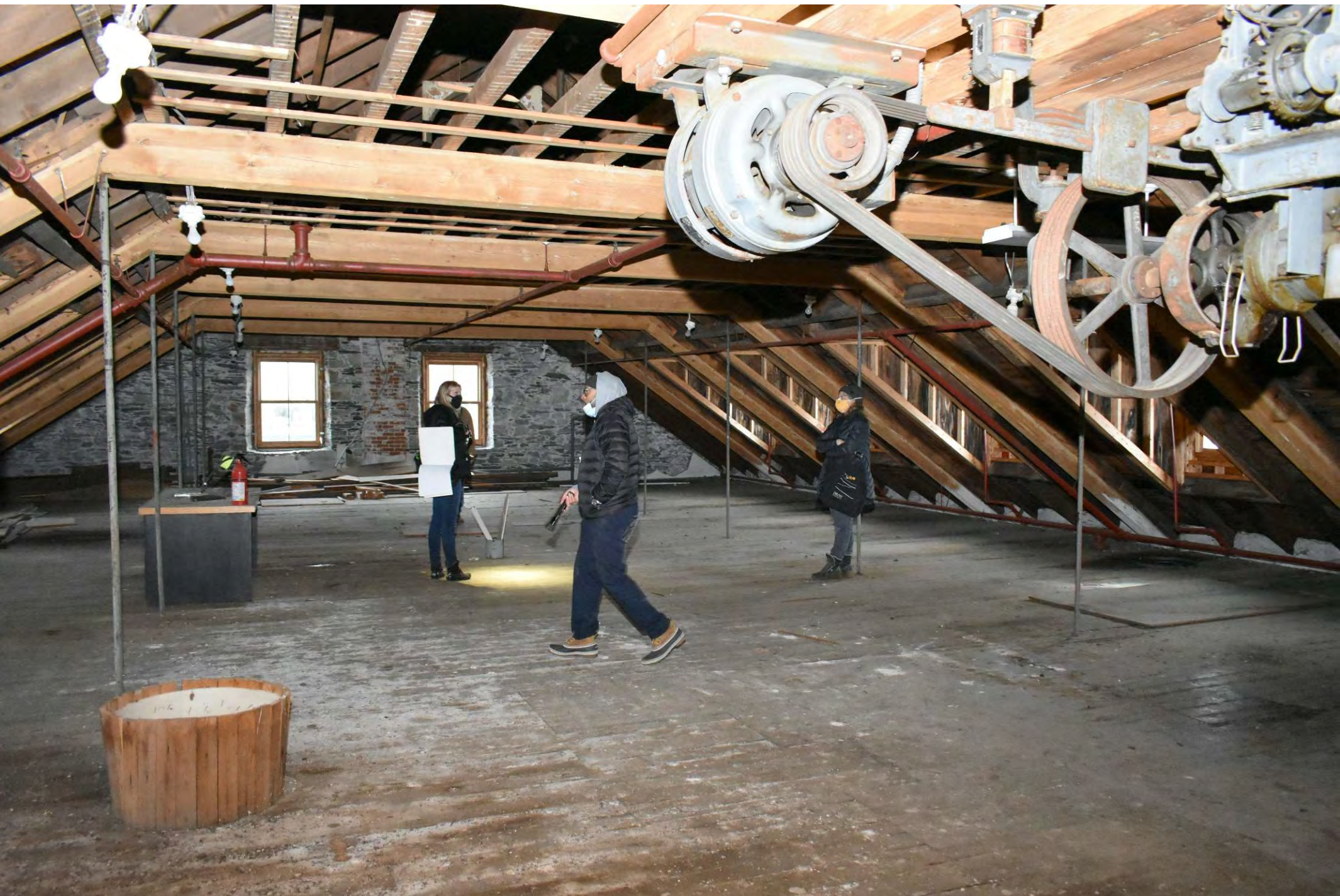
Photo 11 of 30: #4 Mill, attic, facing northeast
