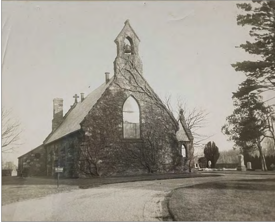
Figure 6 St. Columba's Chapel, view looking southeast, no date.
