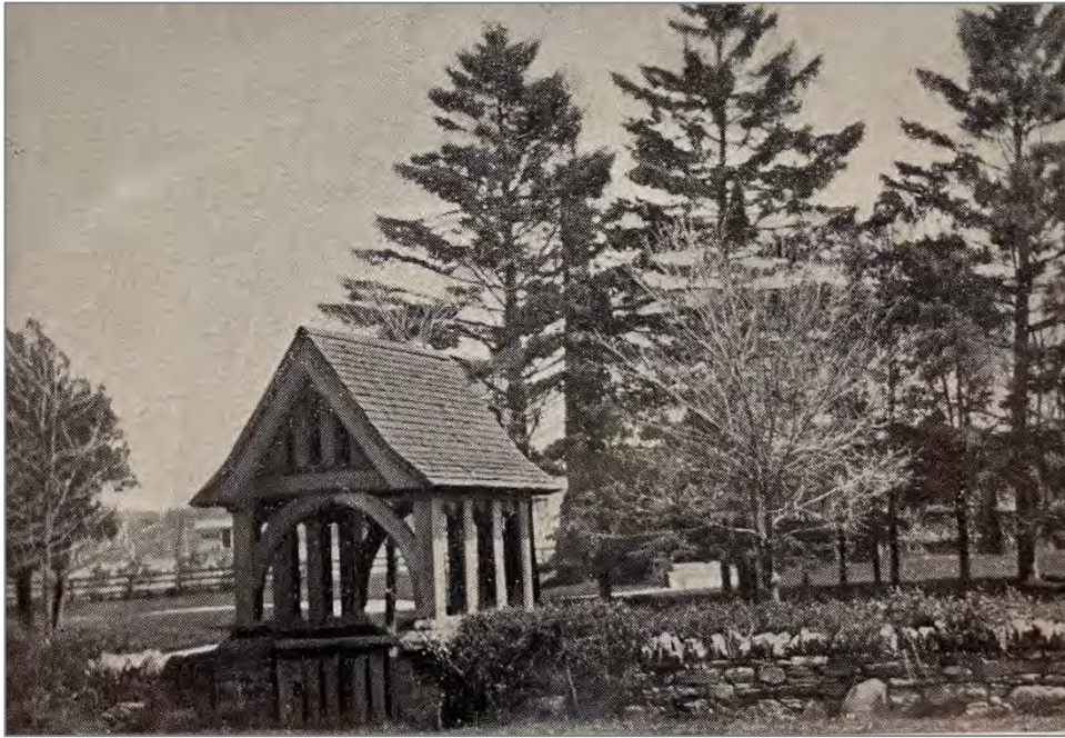
Figure 12 St. Columba's lych gate, view looking north, no date.
