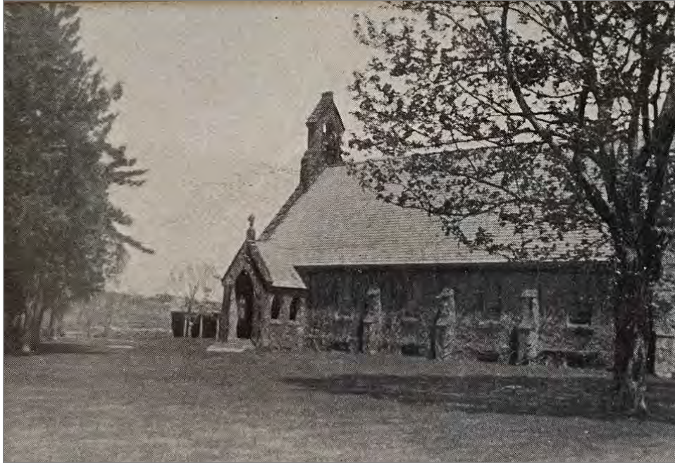
Figure 4 St. Columba's Chapel, view looking northwest, no date.
