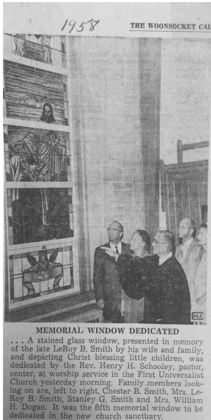
Figure 15 Installation of memorial stained glass window in the addition, 1958. The Woonsocket Call , 1958.
