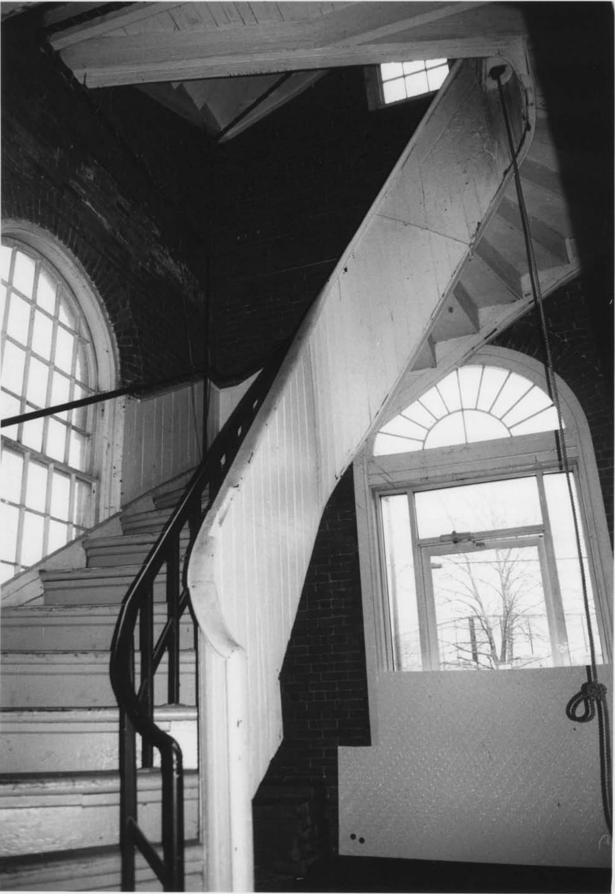
Interior First Floor of Building 1 Stair Tower Rhode Island Tool Company Providence, Providence County, Rhode Island Photograph No. 14
