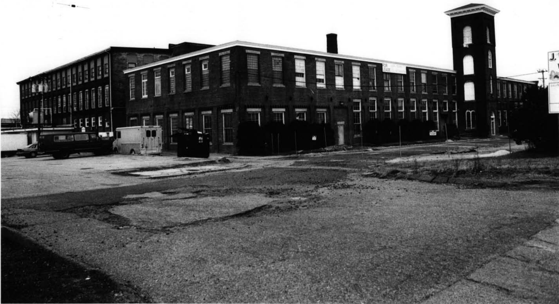
Building II and Building I / Building IA Rhode Island TOOL Company Providence, Providence County, Rhode Island Photograph No. 1
