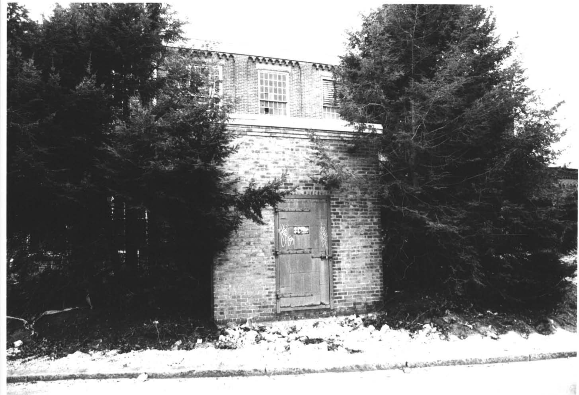
East Elevation of Electrical Substation Rhode Island Tool Company Providence, Providence County, Rhode Island Photograph No. 3
