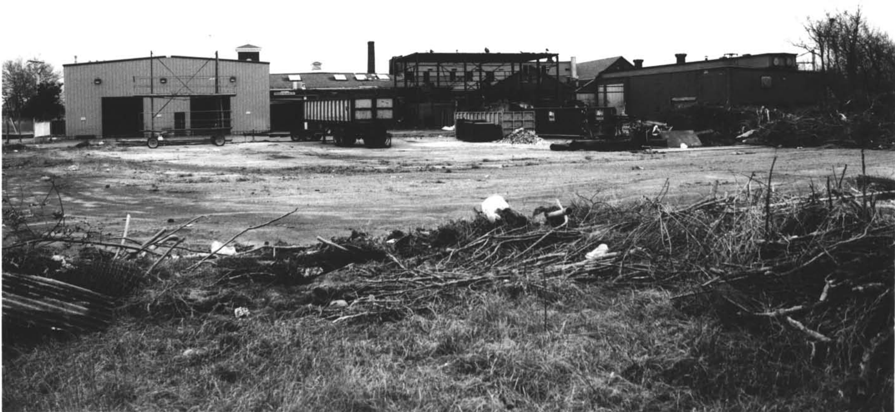
Building 27, Building 26, and Building 22 Rhode Island Tool Company Providence, Providence County, Rhode Island Photograph No. 6
