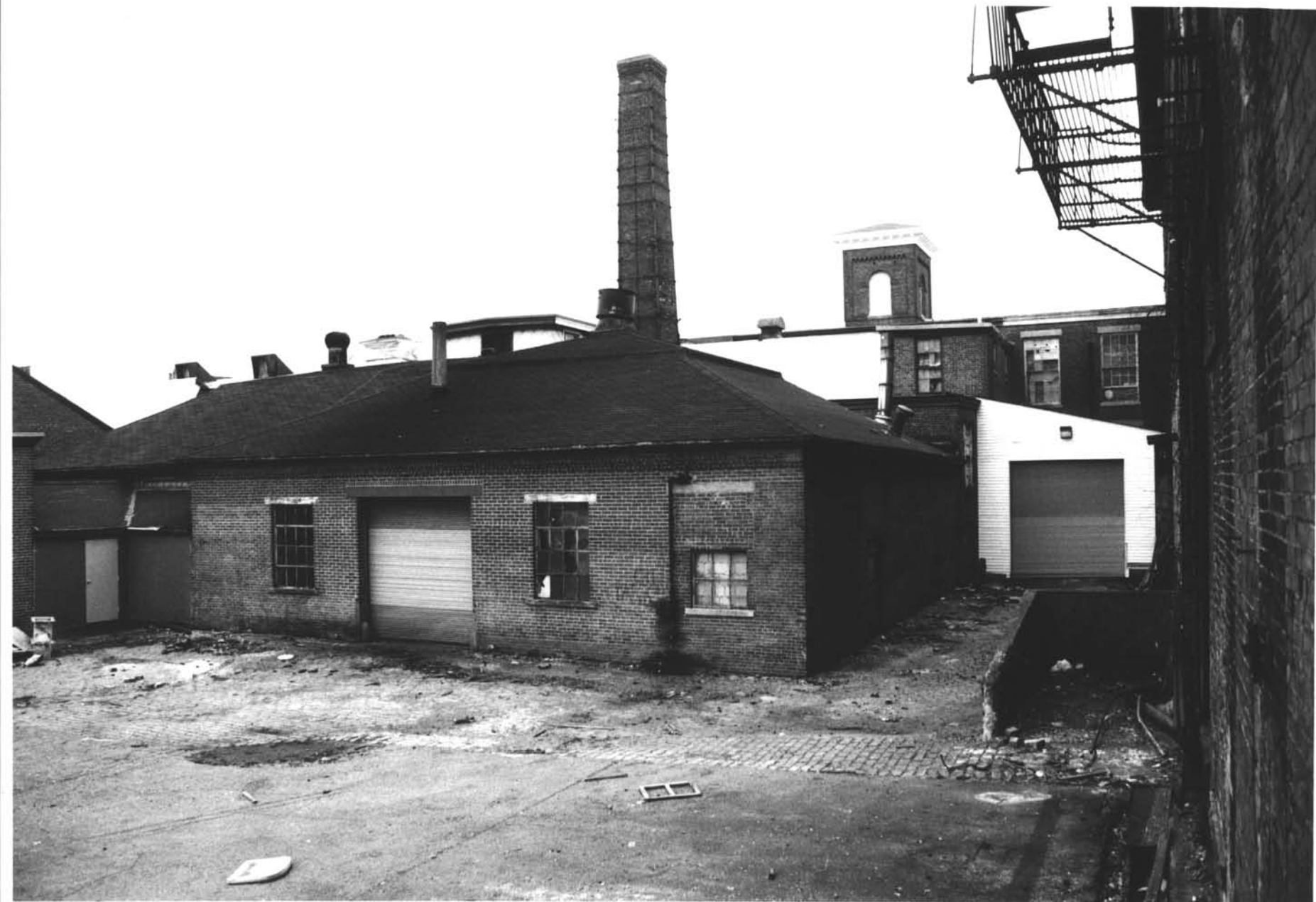
Building 7, Building 6A, And Building 1 Rhode Island Tool Company Providence, Providence County, Rhode Island Photograph No. 12
