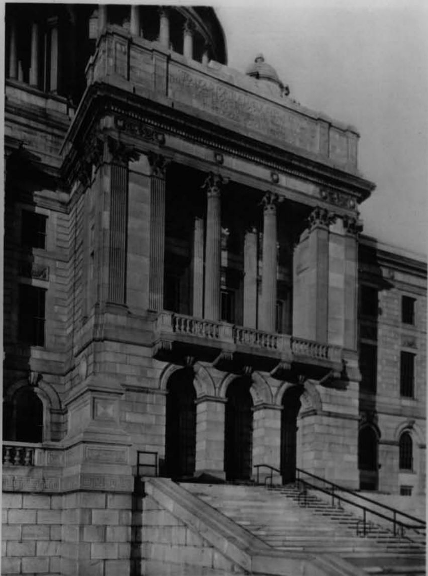
DETAIL OF MAIN ENTRANCE
