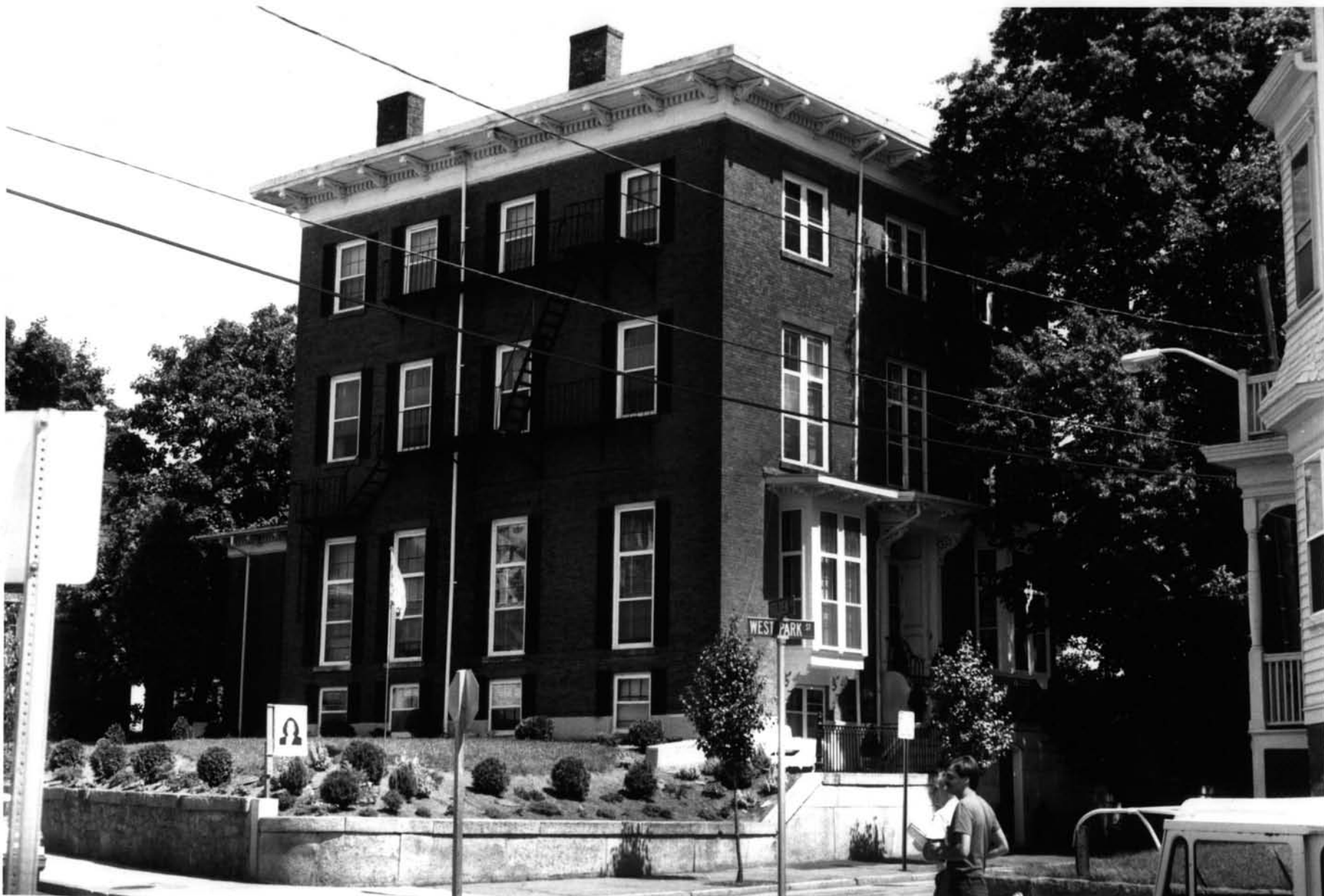
Smith Hill Historic District Providence County Providence, R.I. Photo #8 of 9
