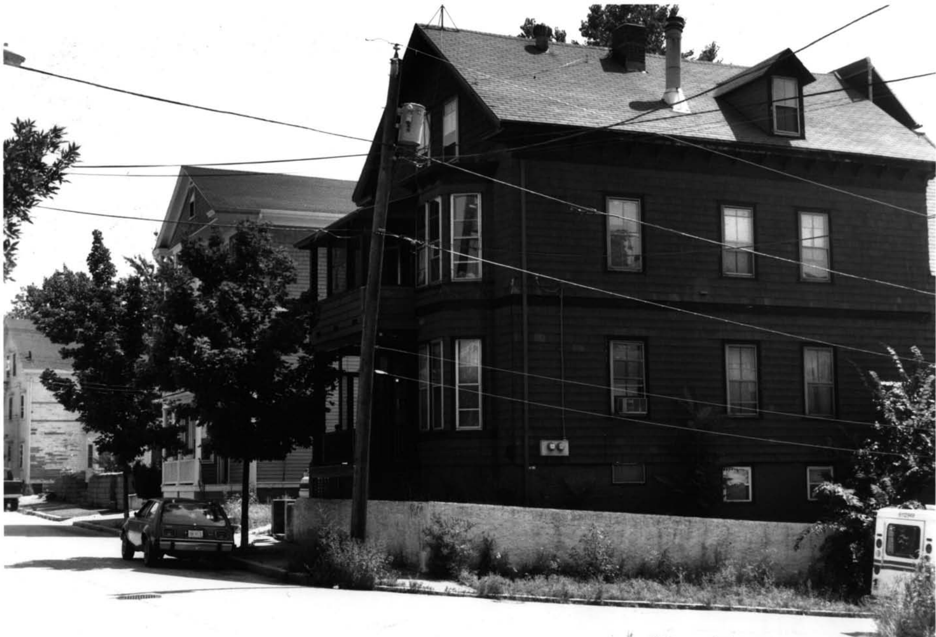
Smith Hill Historic District Providence County Providence, R.I. Photo #7 of 9
