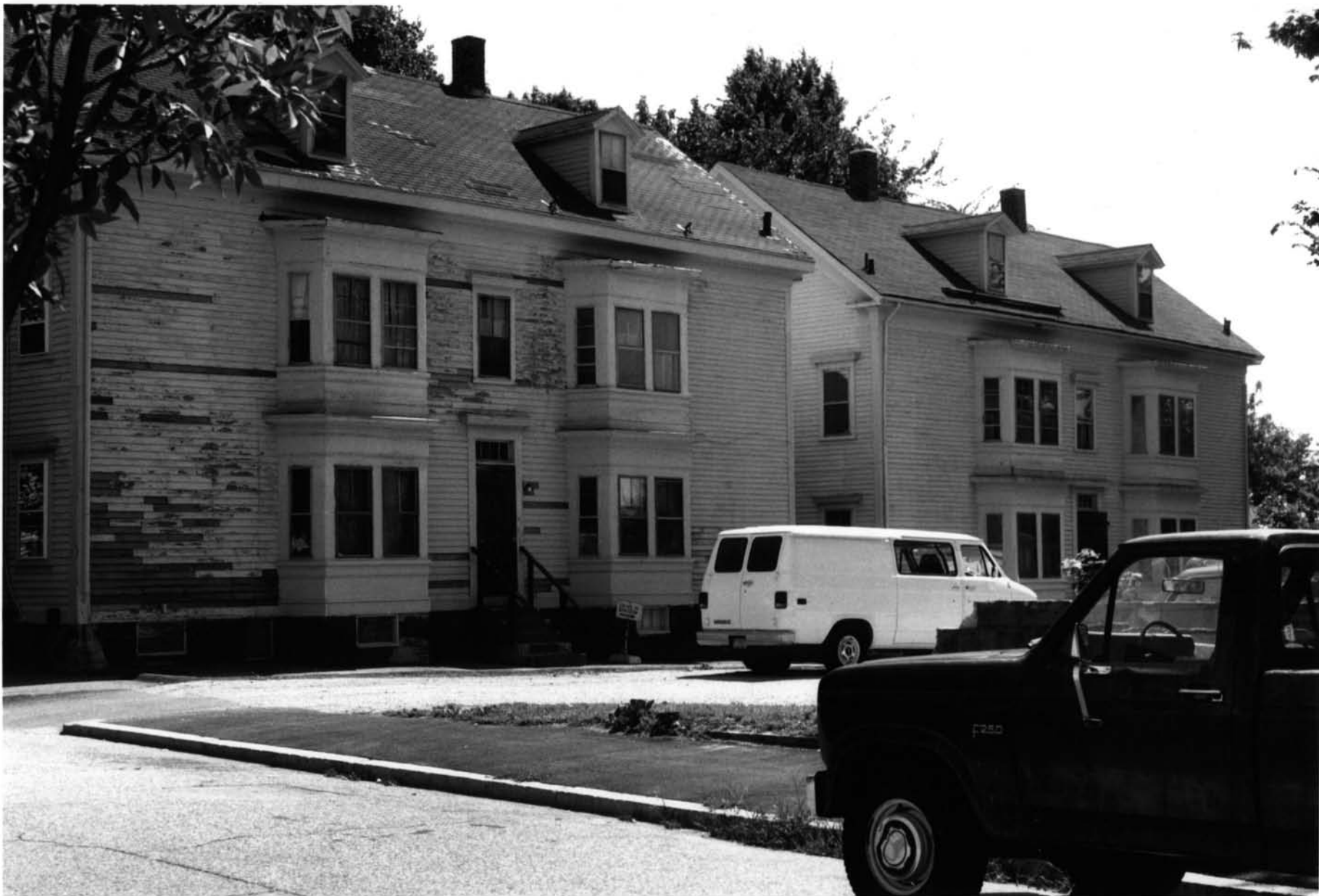
Smith Hill Historic District Providence County Providence, R.I. Photo #6 of 9
