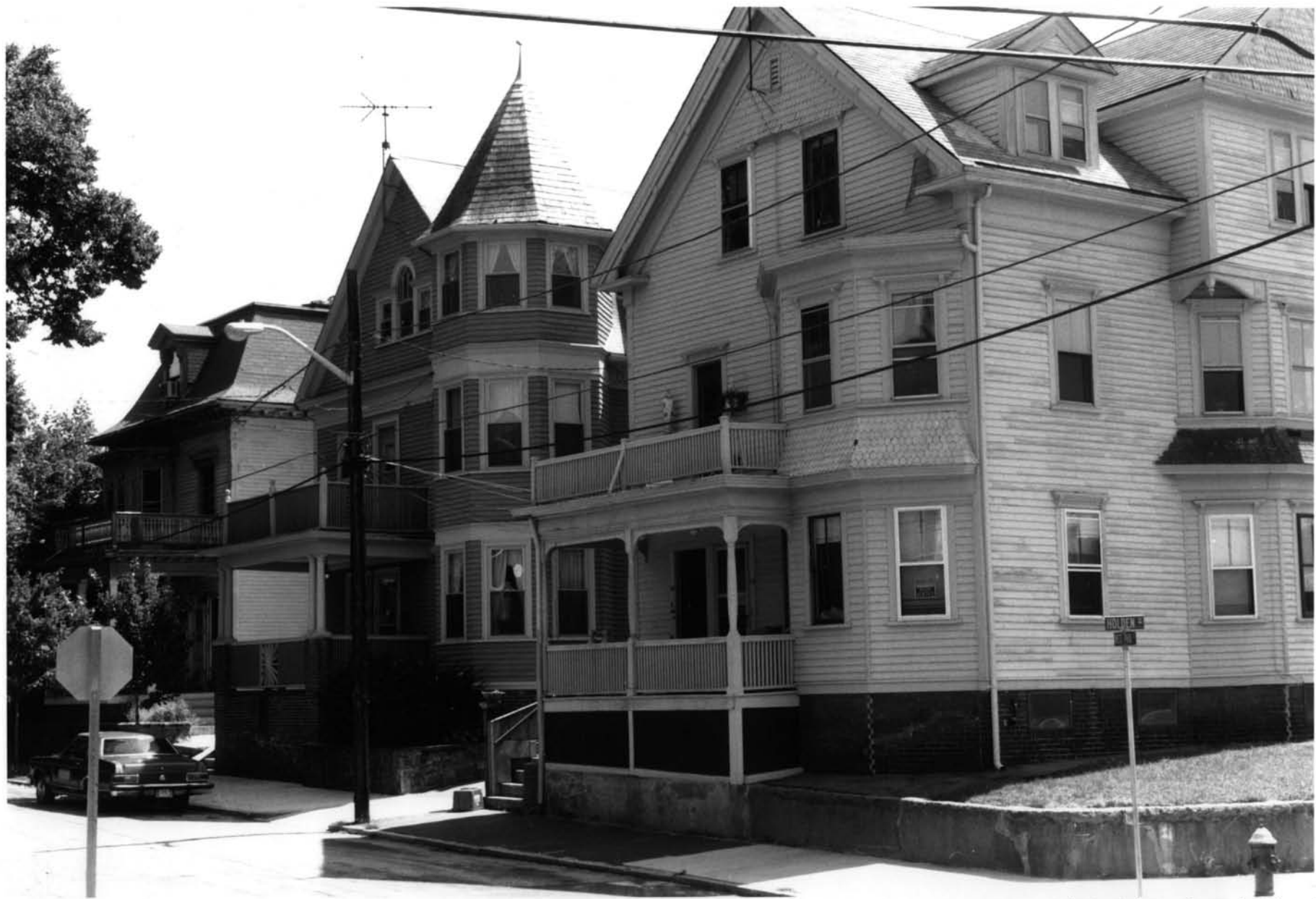
Smith Hill Historic District Providence County Providence, R.I. Photo #9 of 9
