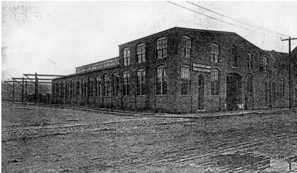
Figure 1 Structural Steel Building (Building 1) View southwest from corner of Sims and Kinsley Avenues 1902
