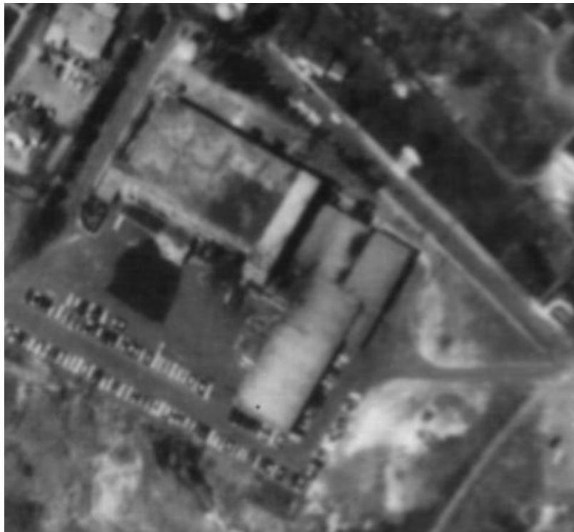
Fig. 5 Rochambeau Worsted Company Mill, 1962 (Aerial Photographs of Providence, RI at http://www.mapper.provplan.org/ha/ )
