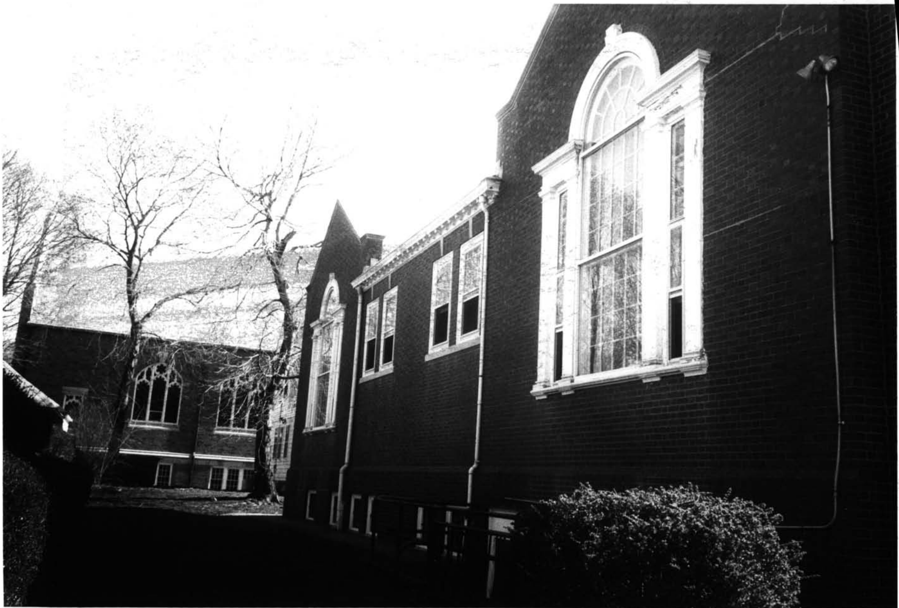
Rochambeau Branch Library Providence City, Prov., R.I. Photo #2 of 3
