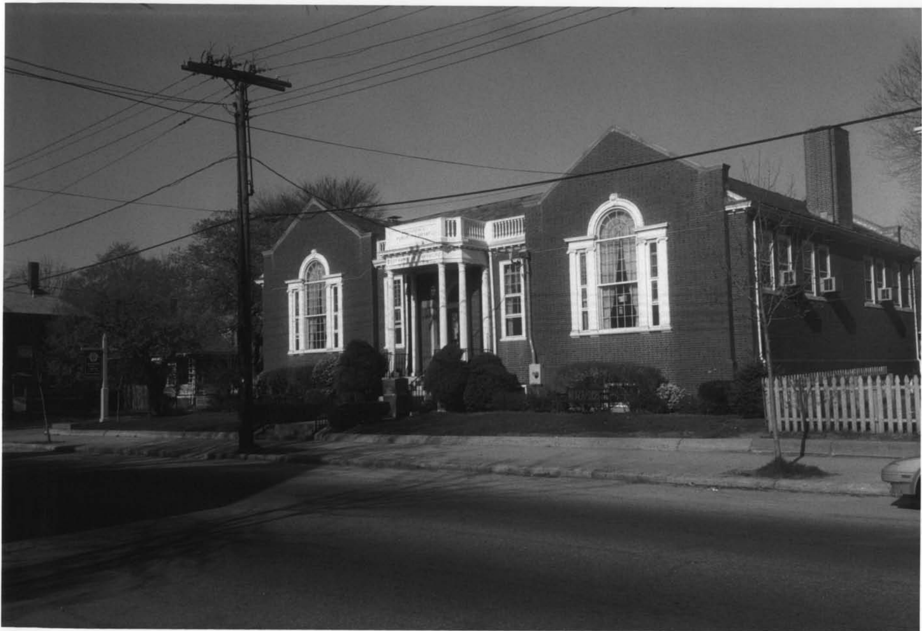
Rochambeau Branch Library Providence City, Prov., R.I. Photo # 1 of 3
