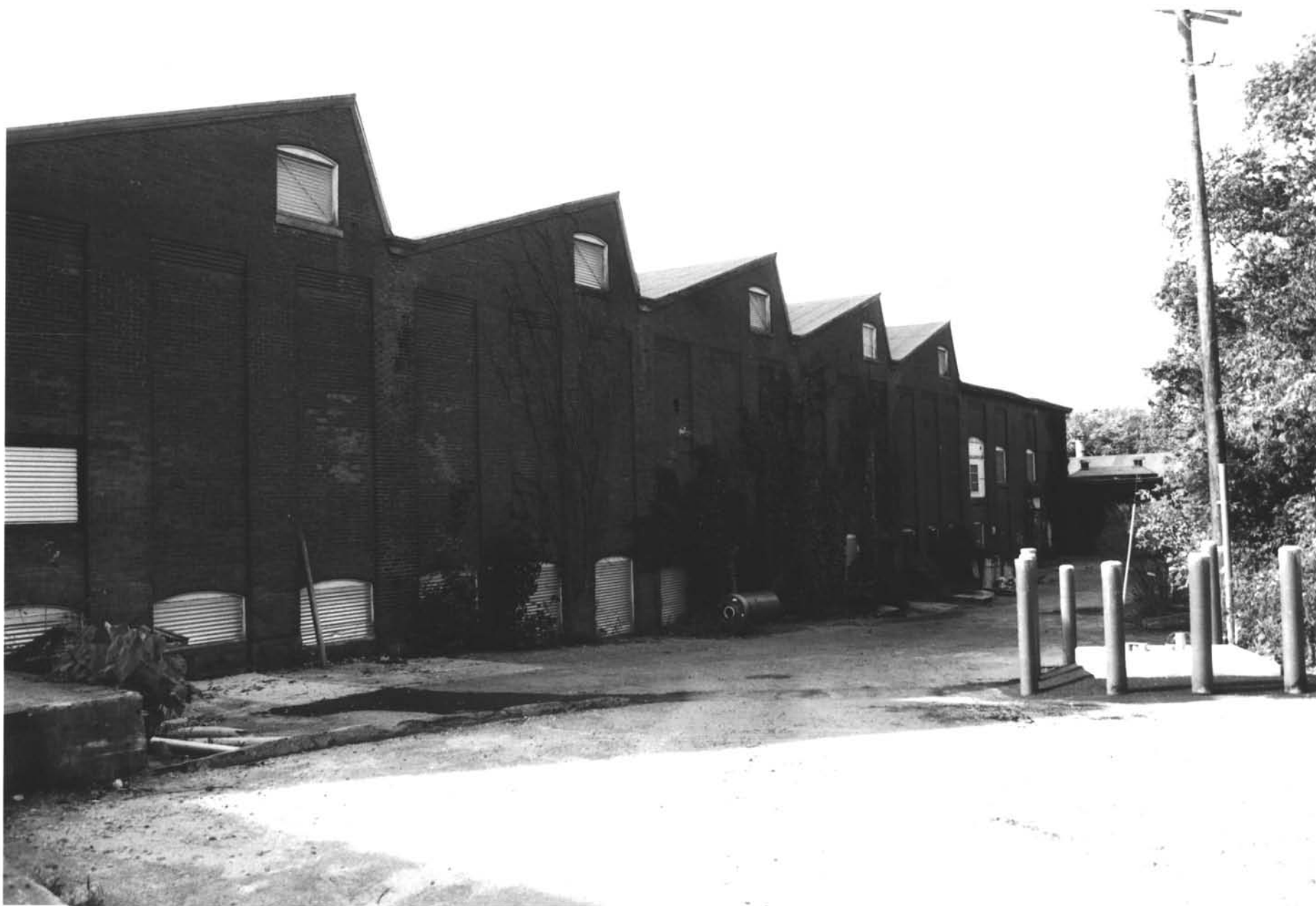
DYE HOUSE WITH WEAVE SHED AT RIGHT GREYSTONE MILL HISTORIC DISTRICT NORTH PROVIDENCE, PROVIDENCE COUNTY RHODE ISLAND PHOTOGRAPH NUMBER 6
