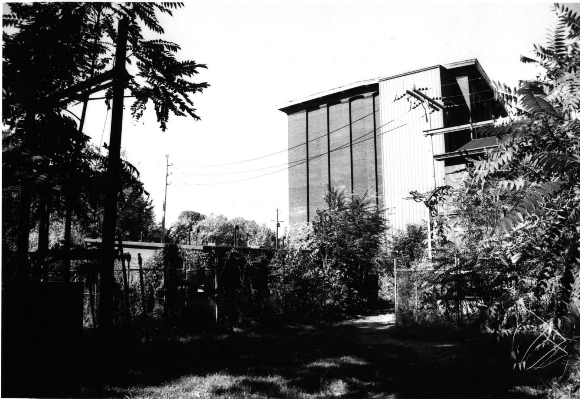
OIL HOUSE, MAIN MILL AND DYE HOUSE GREYSTONE MILL HISTORIC DISTRICT NORTH PROVIDENCE, PROVIDENCE COUNTY RHODE ISLAND PHOTOGRAPH NUMBER 9
