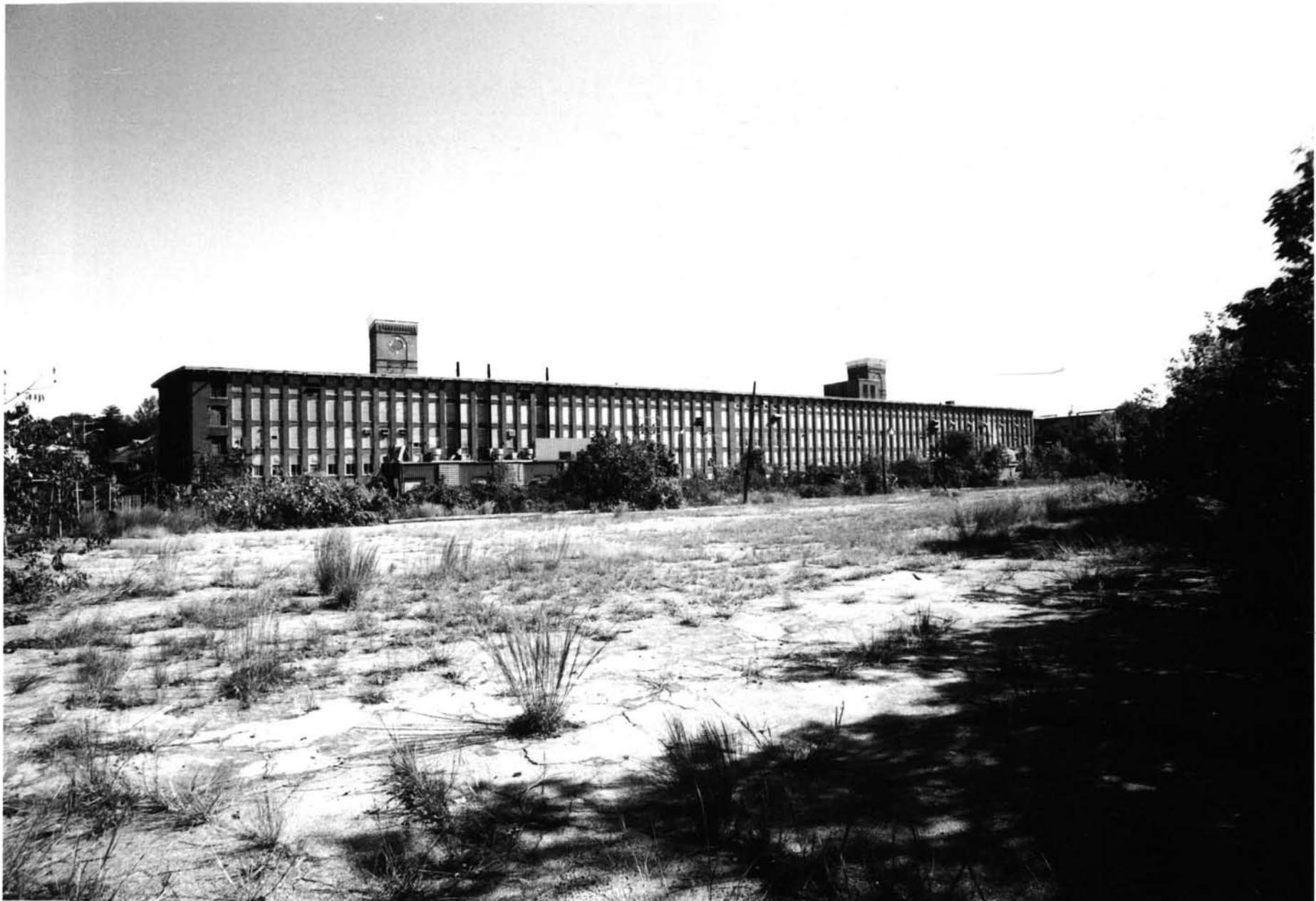
WEST ELEVATION OF MAIN MILL GREYSTONE MILL HISTORIC DISTRICT NORTH PROVIDENCE, PROVIDENCE COUNTY, RHODE ISLAND PHOTOGRAPH NUMBER 1
