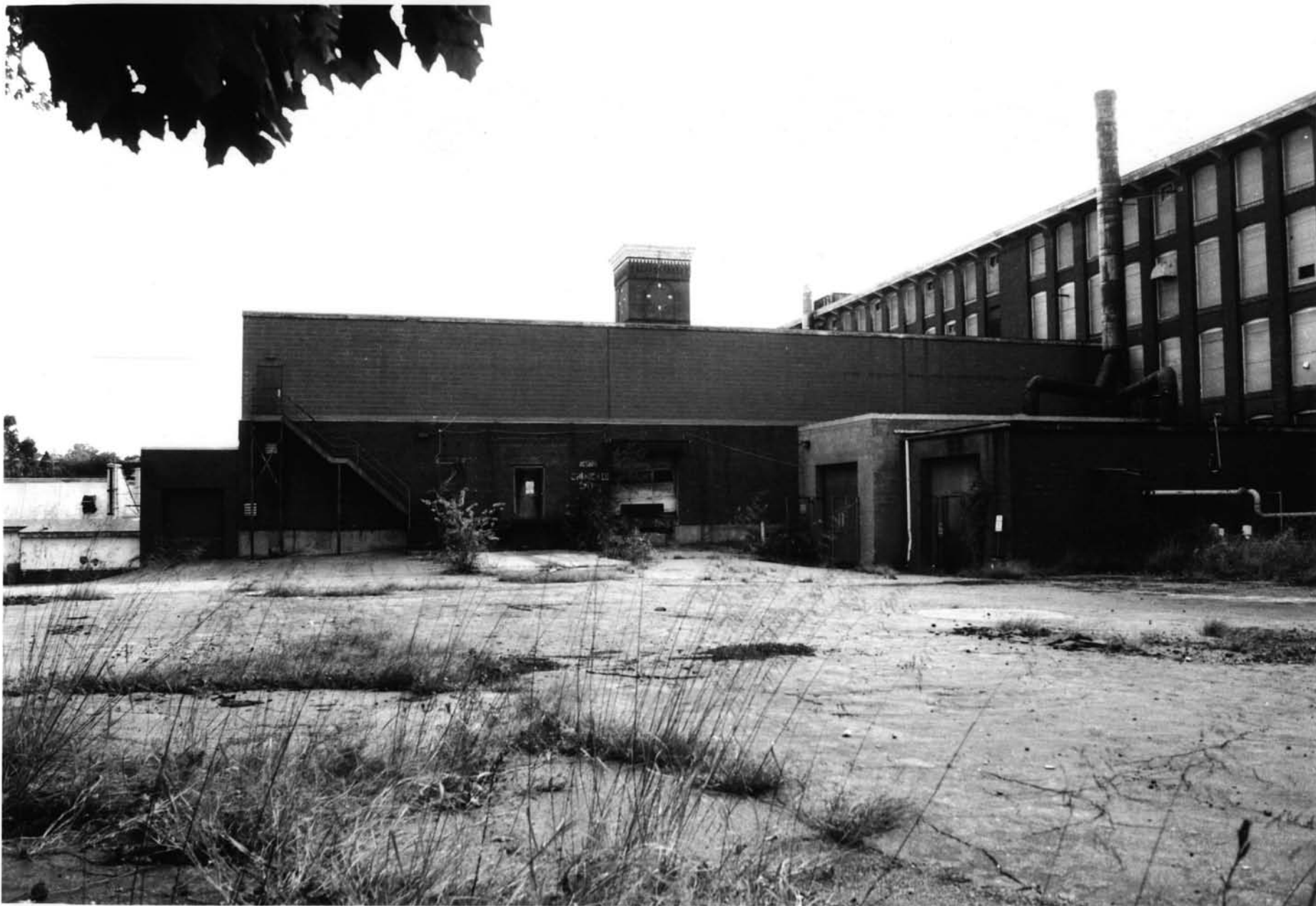
Weave Shed and Main Mill Greystone Mill Historic District North Providence, Providence County Rhode Island Photograph Number 3
