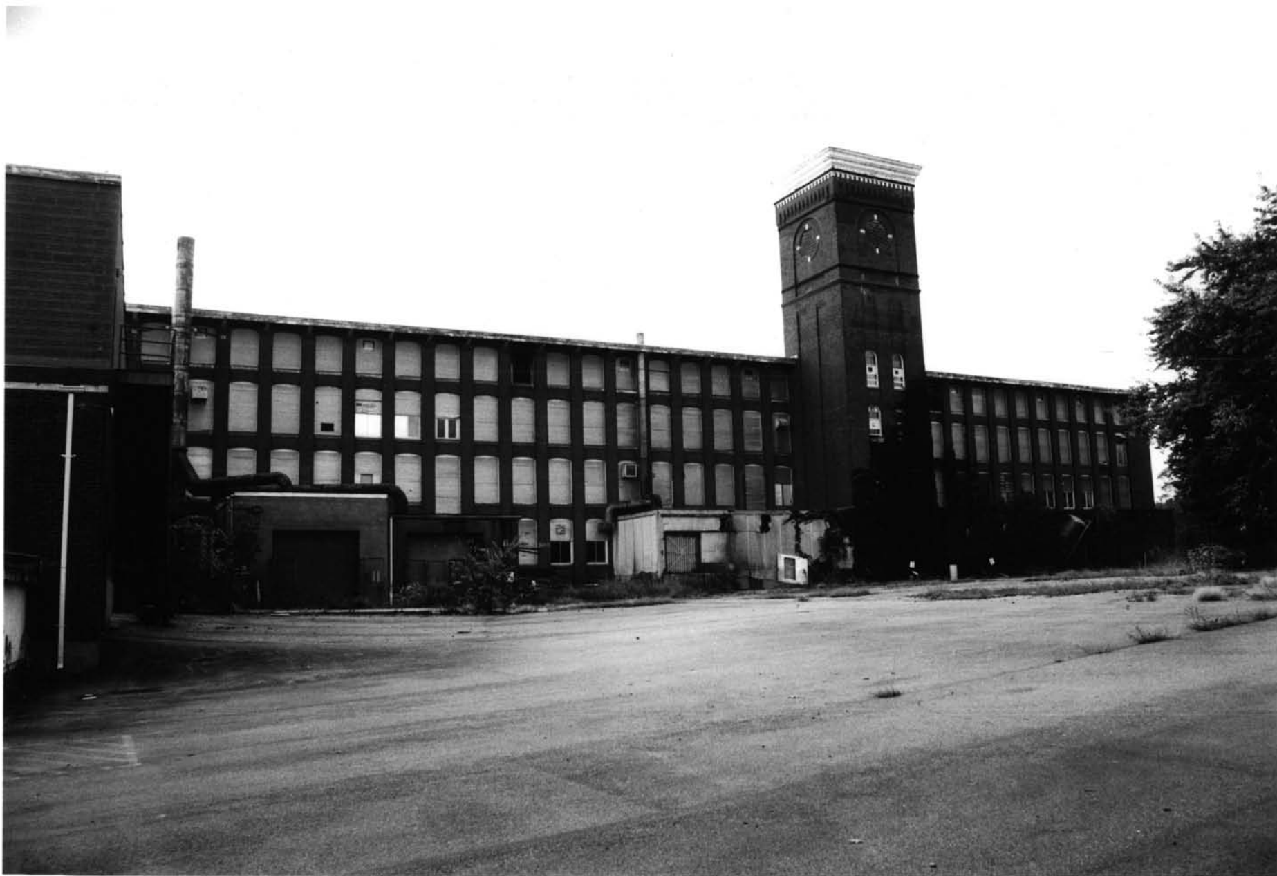
Main Mill and North Tower Greystone Mill Historic District North Providence, Providence County Rhode Island Photograph Number 4
