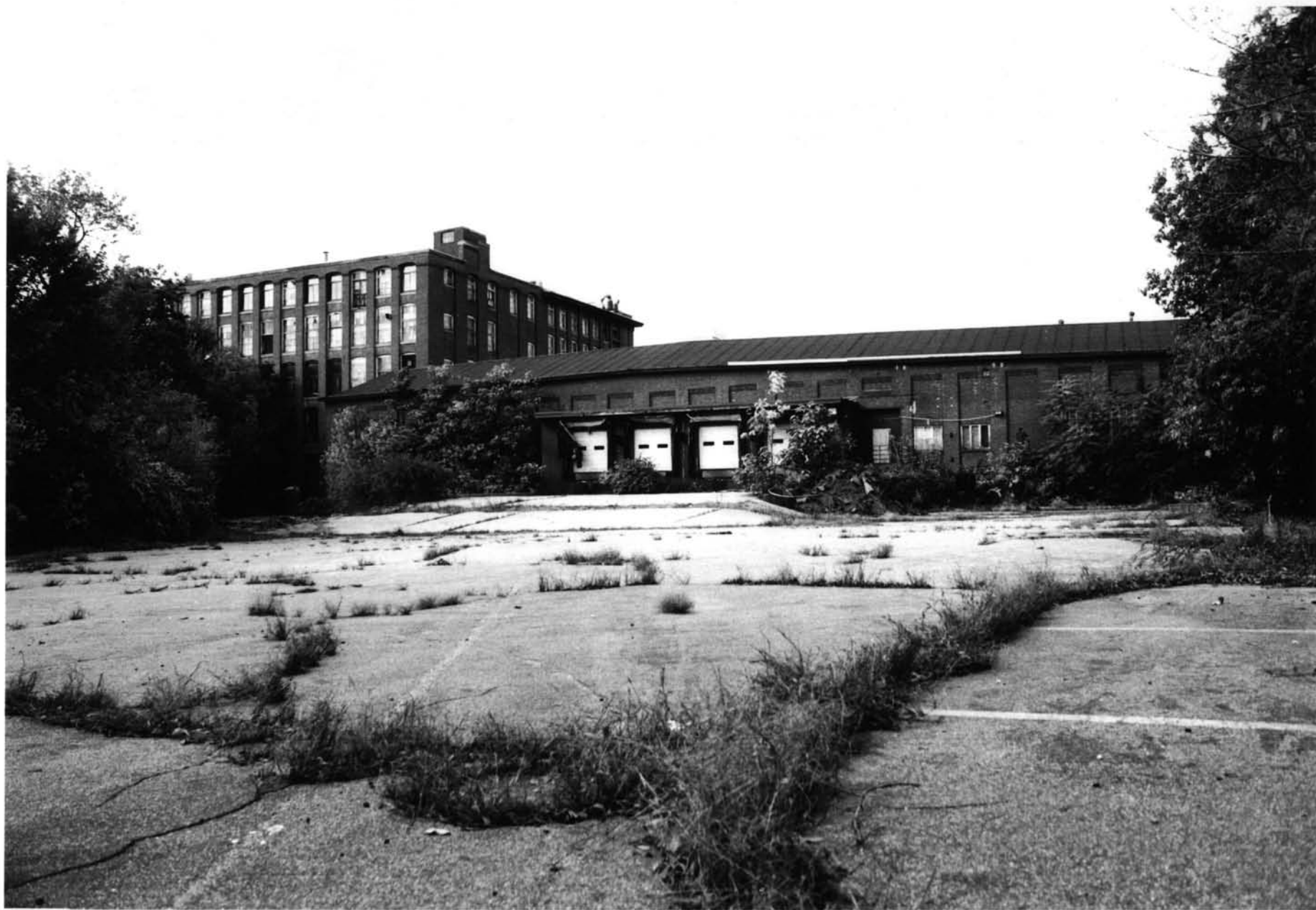
FINISHING BUILDING AND DYE HOUSE GREYSTONE MILL HISTORIC DISTRICT NORTH PROVIDENCE, PROVIDENCE COUNTY RHODE ISLAND PHOTOGRAPH NUMBER 7
