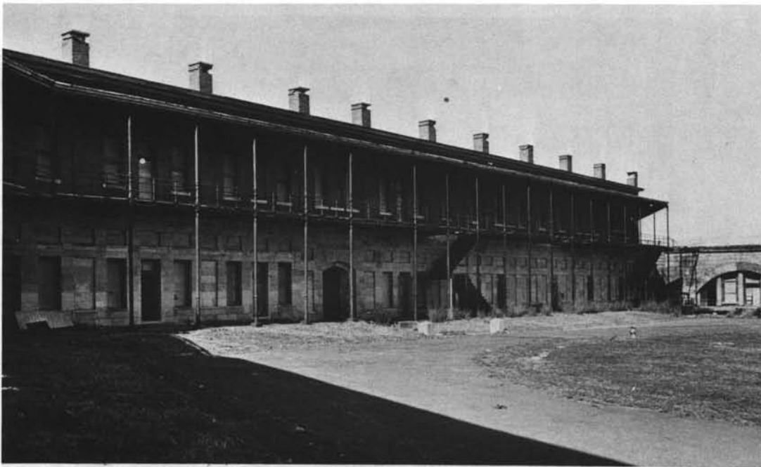
Main Work, Fort Adams Newport, Rhode Island
