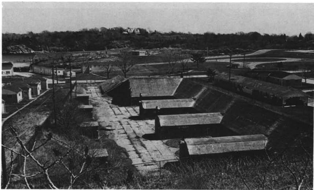
Batteries, Fort Adams Newport, Rhode Island April 1975 Photo: AASLH
