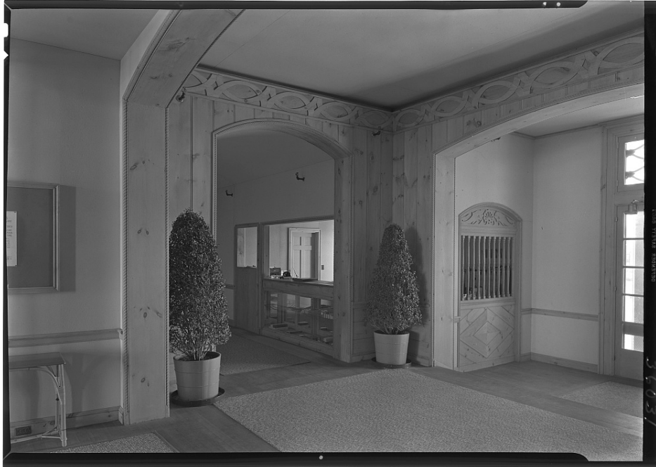
Photo 4 of 5 The Dunes Club, view of clubhouse interior, lobby, looking northwest, 1939.
