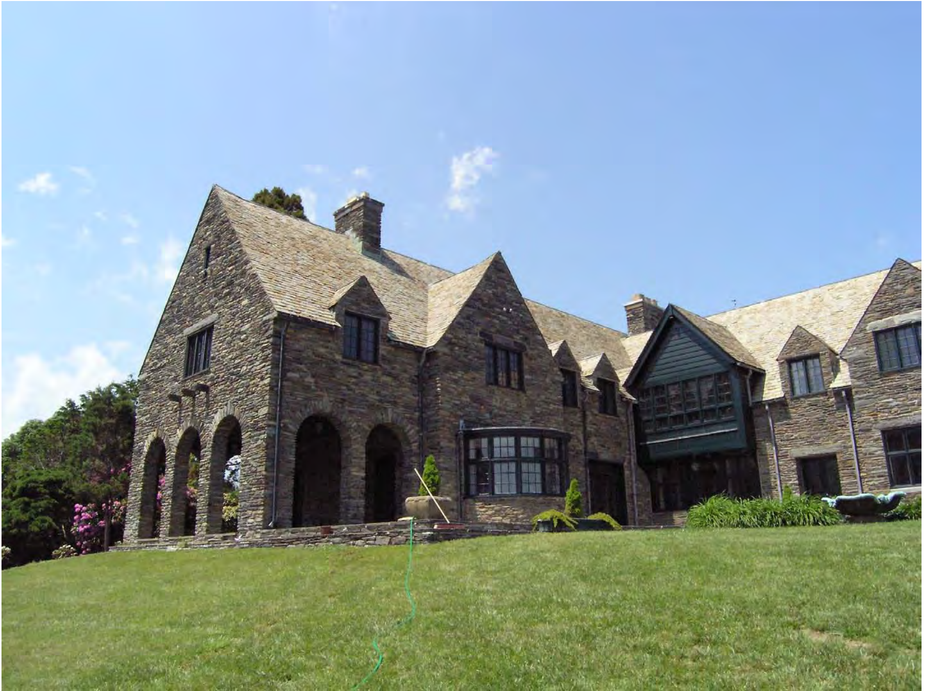
501 Indian Avenue, Middletown, RI Stonybrook Southeast elevation
