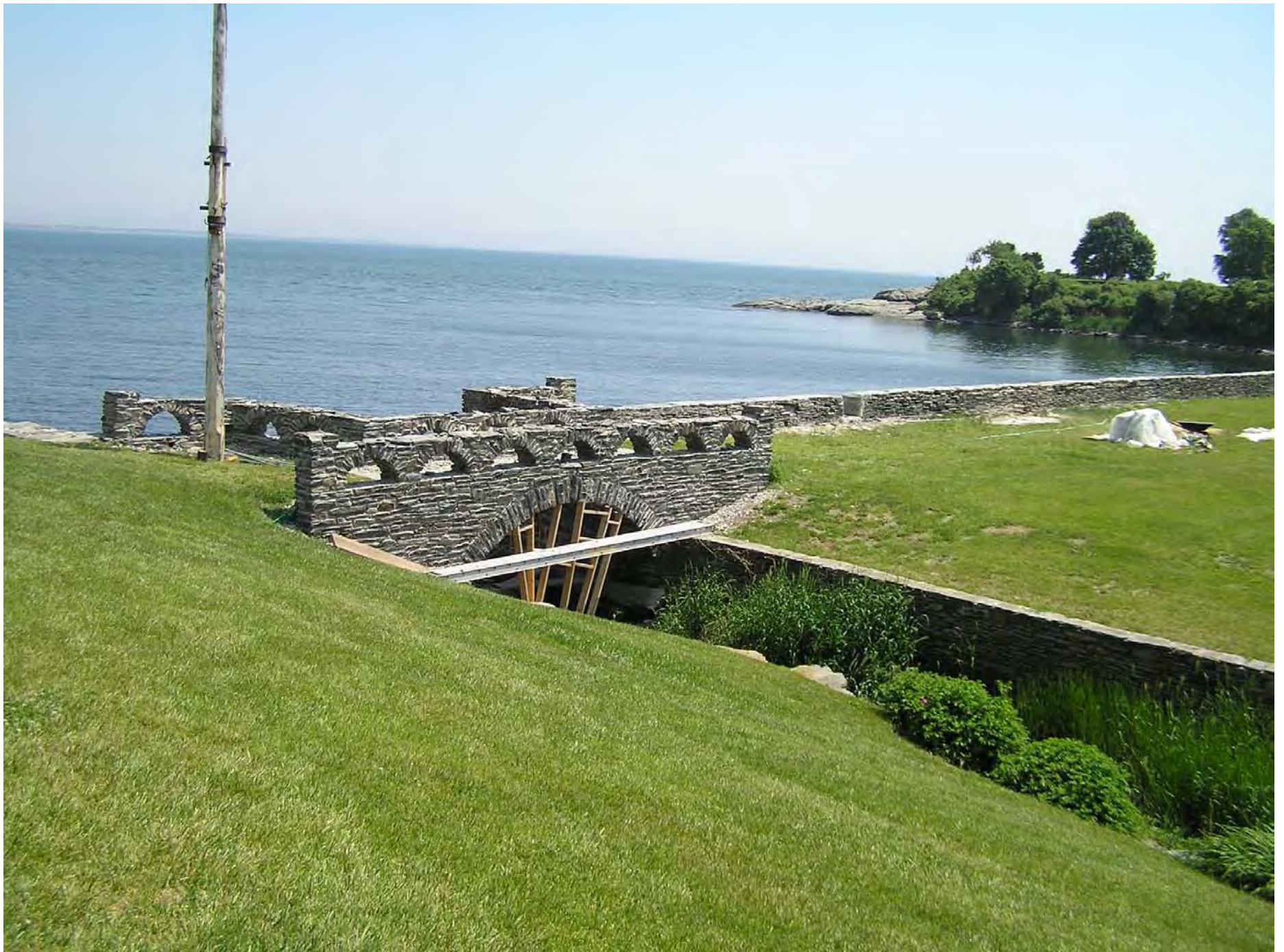
501 Indian Avenue, Middletown, RI Stonybrook – stone bridge Looking southeast
