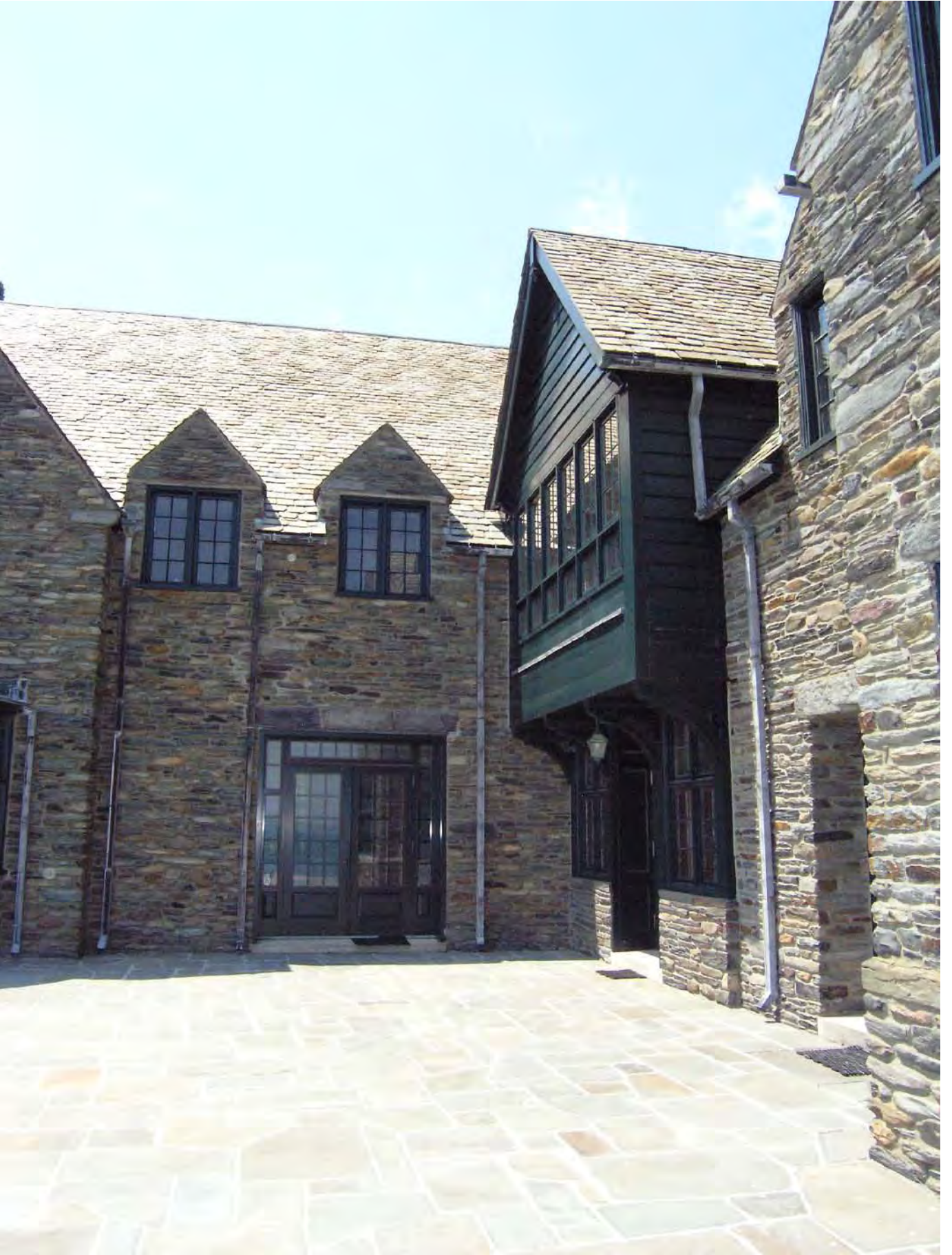
501 Indian Avenue, Middletown, RI Stonybrook – entrance detail Southeast elevation
