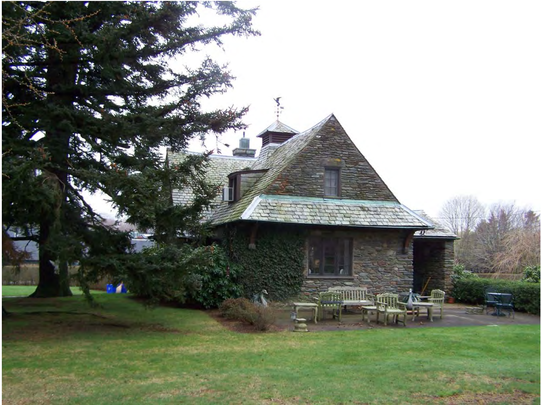
75 Vaucluse Avenue, Indian Avenue, Middletown, RI Stonybrook Gardener's Cottage Northeast elevation
