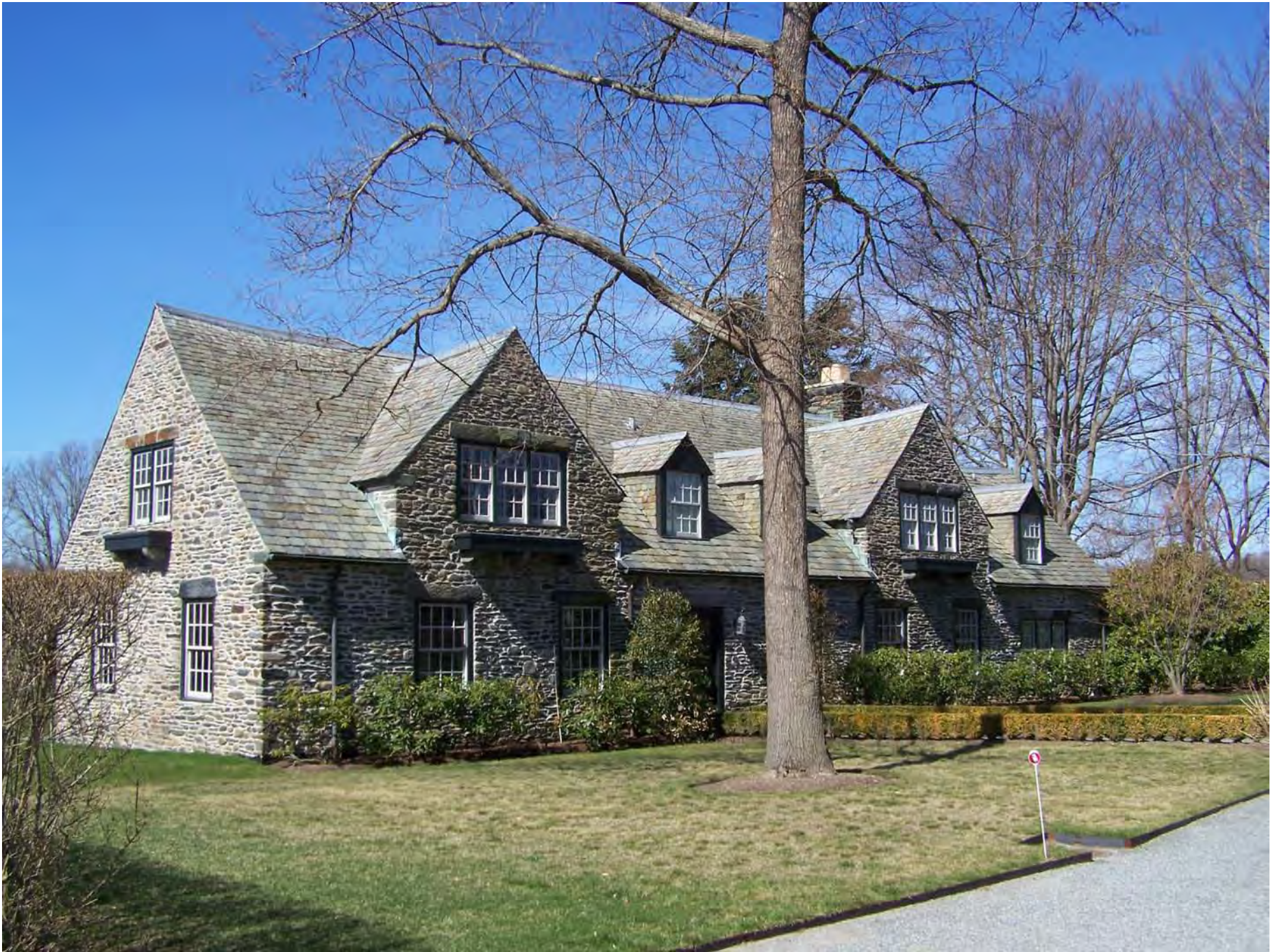
502 Indian Avenue, Middletown, RI Stonybrook Carriage House Northeast elevation
