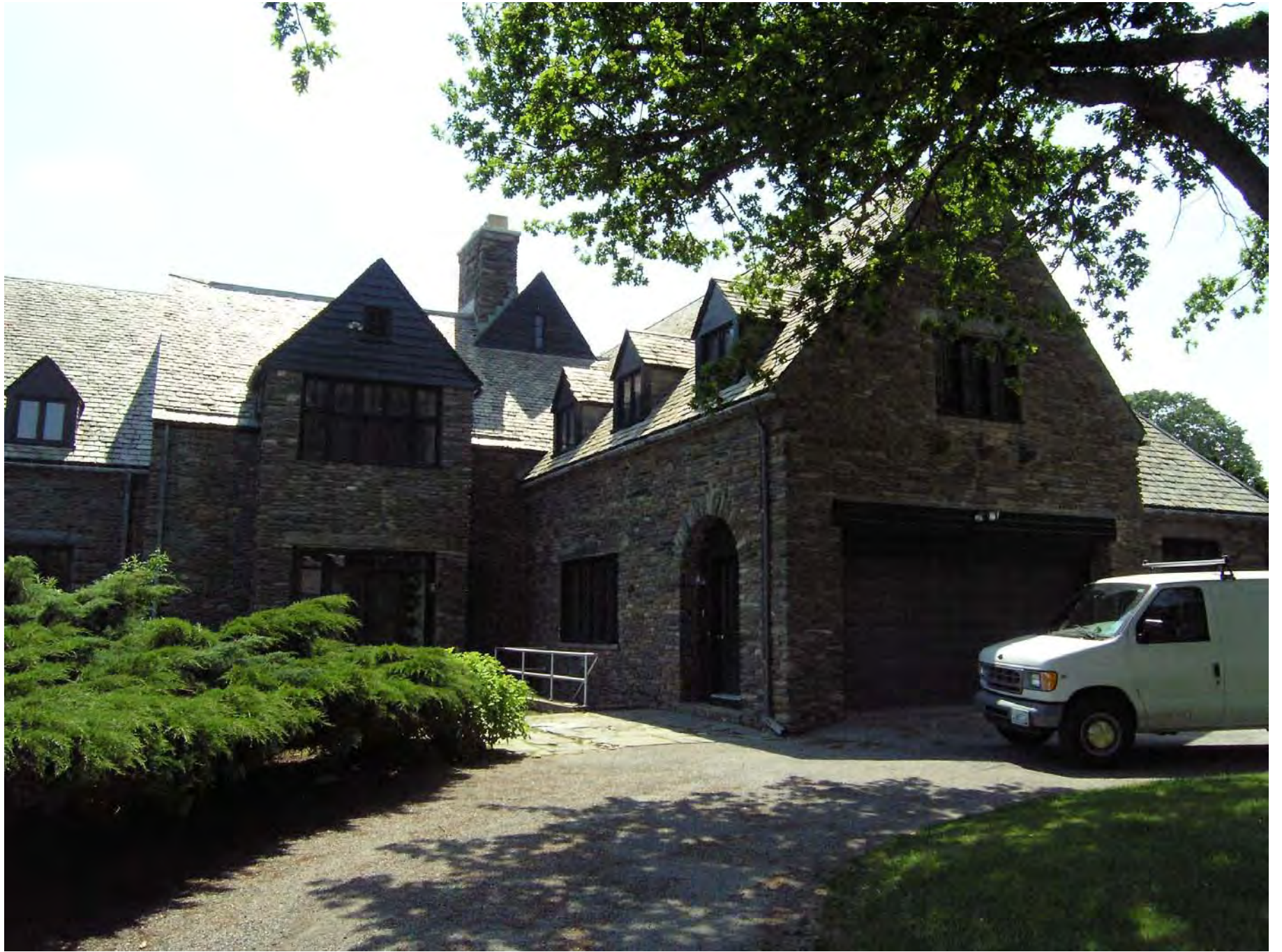
501 Indian Avenue, Middletown, RI Stonybrook – entrance and garage Northeast elevation
