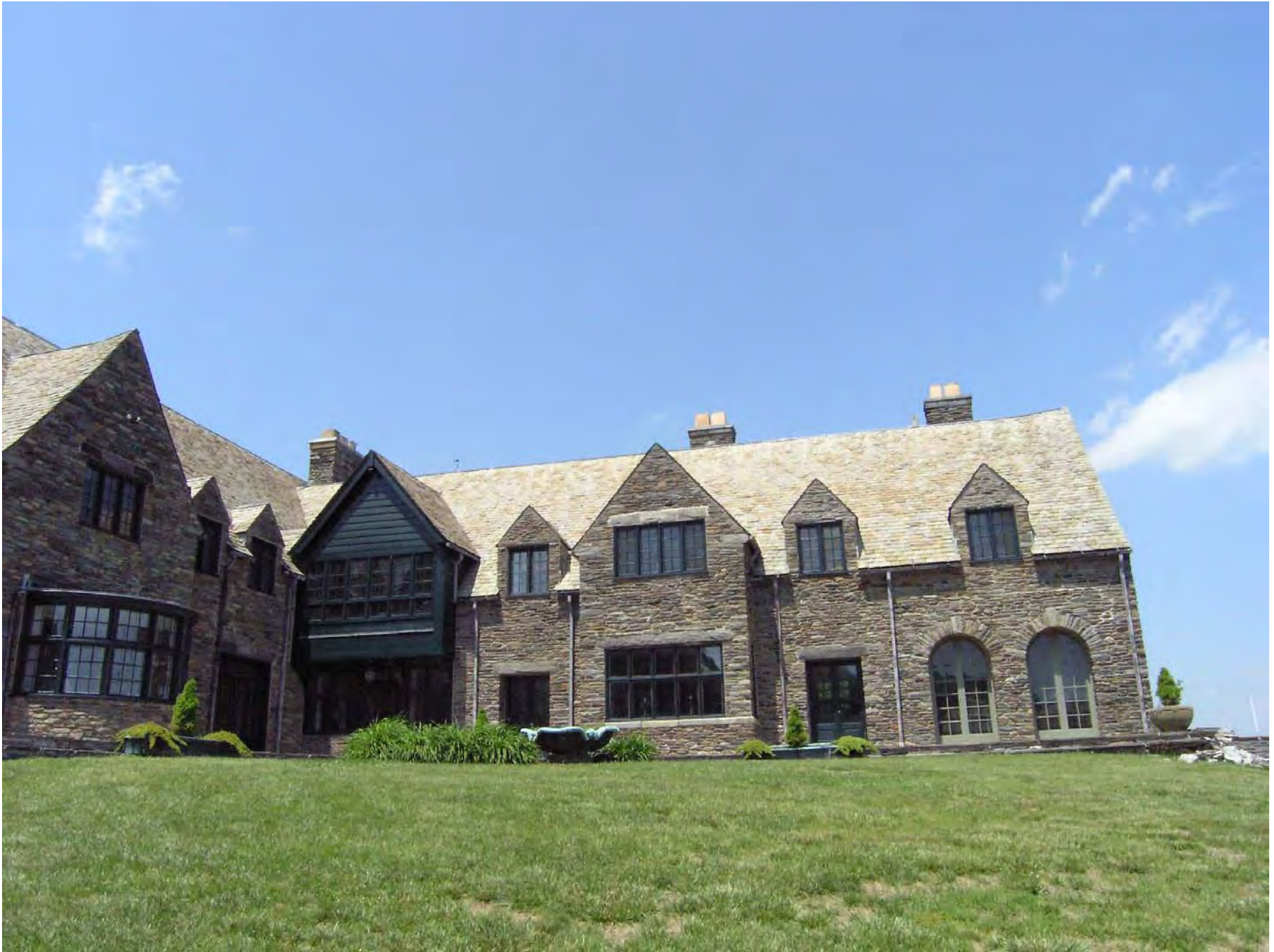
501 Indian Avenue, Middletown, RI Stonybrook Southeast elevation
