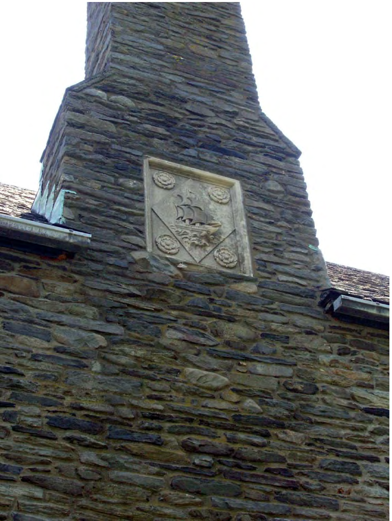
501 Indian Avenue, Middletown, RI Stonybrook – chimney detail Northeast elevation
